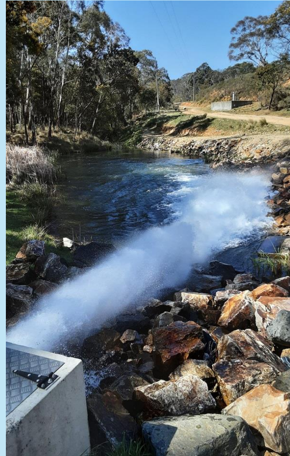
Thompsons Creek Reservoir discharge into Thompsons Creek 30 September 2023
