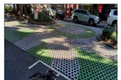
Traffic calming pavement treatment- The Corso, Manly. Suggested use to highlight focal points, intersections and way-finding.
