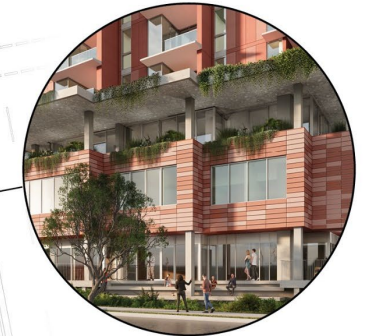
Stepped transition along Harris St
