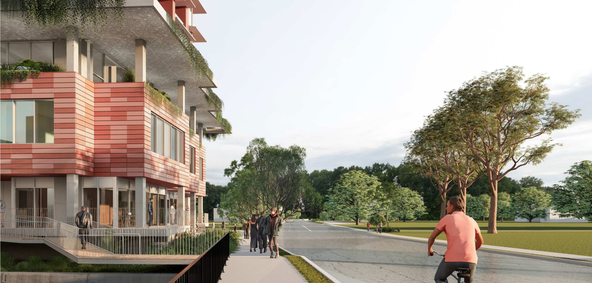
Harris St – Clay Cliff Creek Frontage
