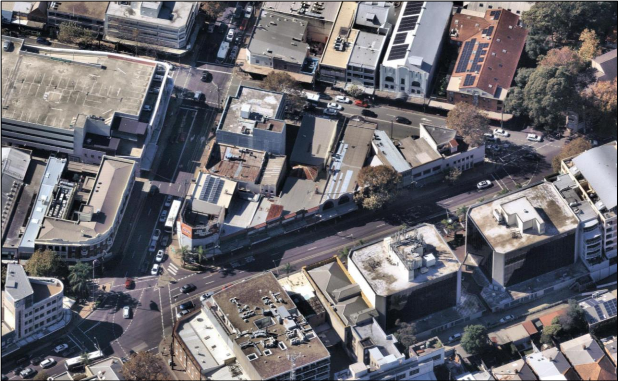
Figure 3 Existing development on the site viewing the Pacific Highway frontage (Source: nearmap )
