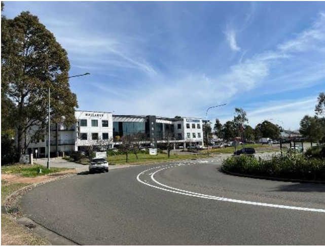
Site frontage to Brookhollow Avenue, looking north-west
