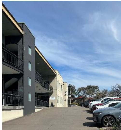
Existing commercial building and carpark on Site, looking west
