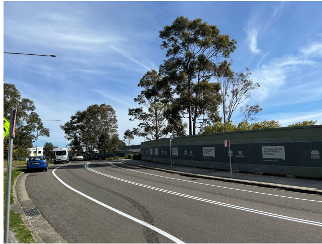
Brookhollow Avenue and rear of Norwest Metro Station, looking north-west
