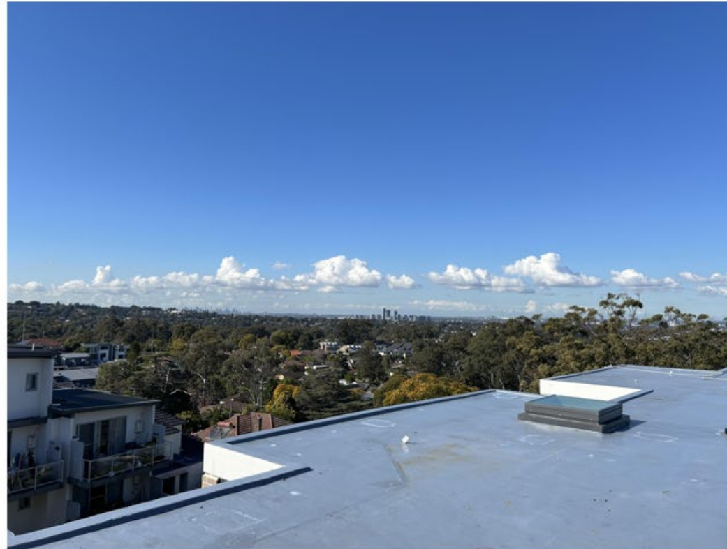
Looking southeast across the northeast corner of the project site
