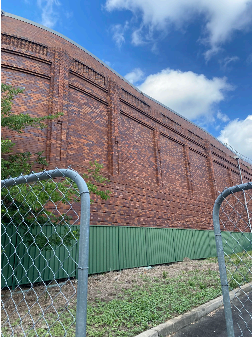
Image 2 – View of Sydney Water Reservoir
