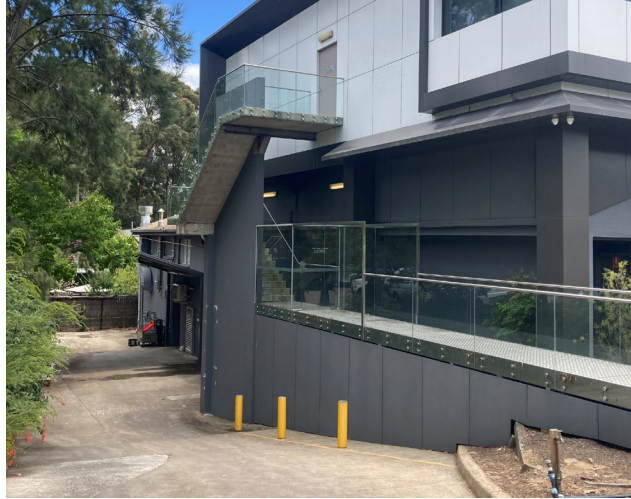
View of connection point between Stage 1 and 2 buildings and existing loading access.
