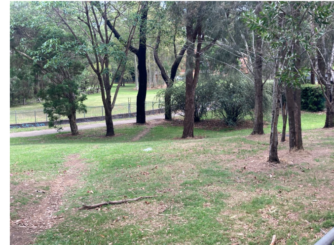
View of Lytton Street Park and Finlaysons Creek culvert, looking north-west.
