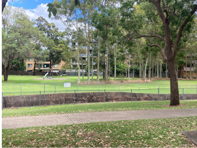
View of Lytton Street Park and Finlaysons Creek culvert, looking west.
