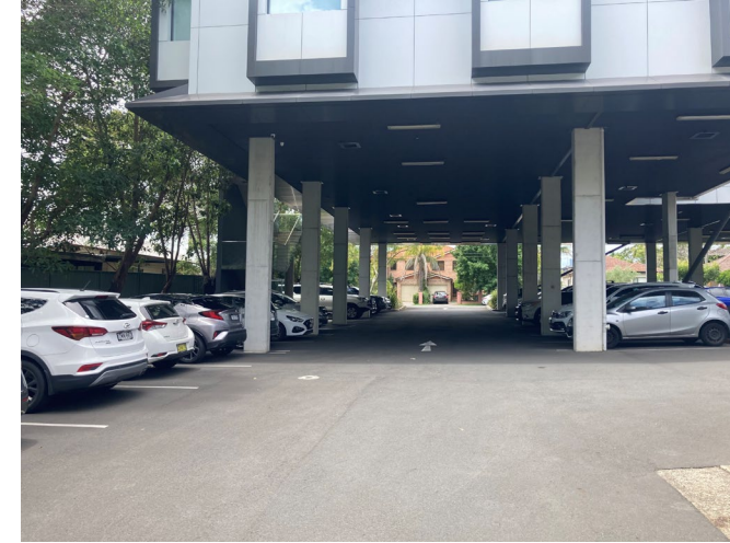
View of rear of undercroft area, existing carpark, and flood levels looking east.
