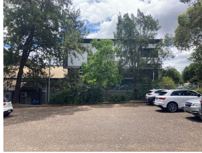
View of connection point from within southern carpark, looking north.
