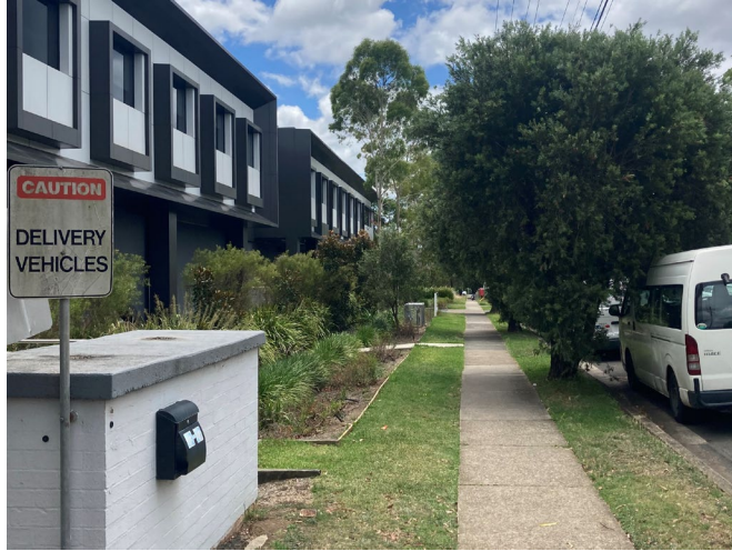
View of site frontage to Lytton Street, looking north.
