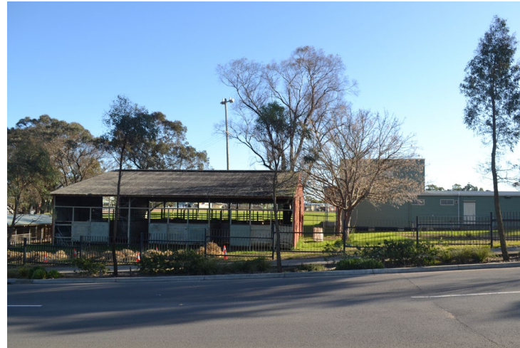
View of The Hills Showground looking north from De Clambe Drive with showground buildings in the foreground.
