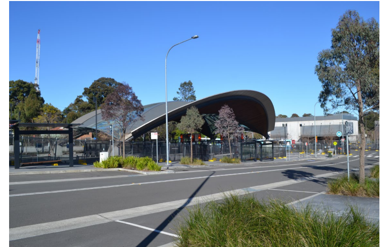
View of the Hills Showground Metro Station looking south-west from Mandala Parade.
