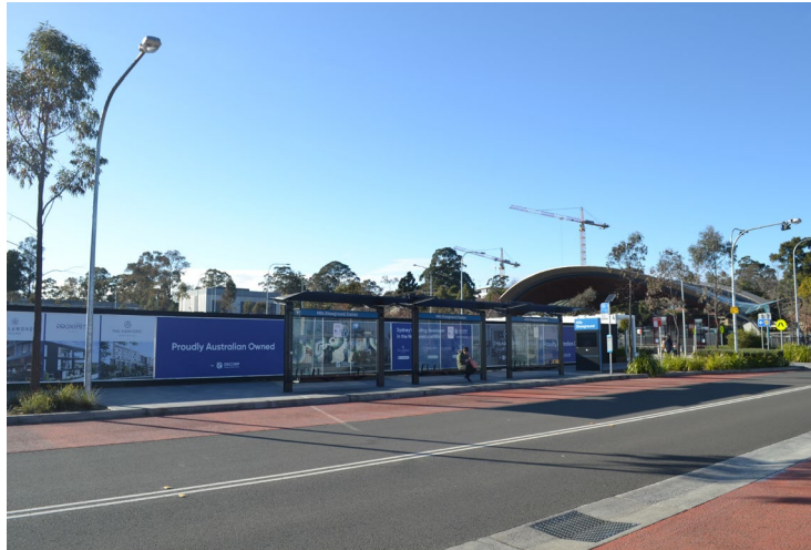
View of the site looking south-east, including the Hills Showground Metro Station beyond.
