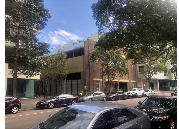
Neild Ave, view NNW to No. 10
