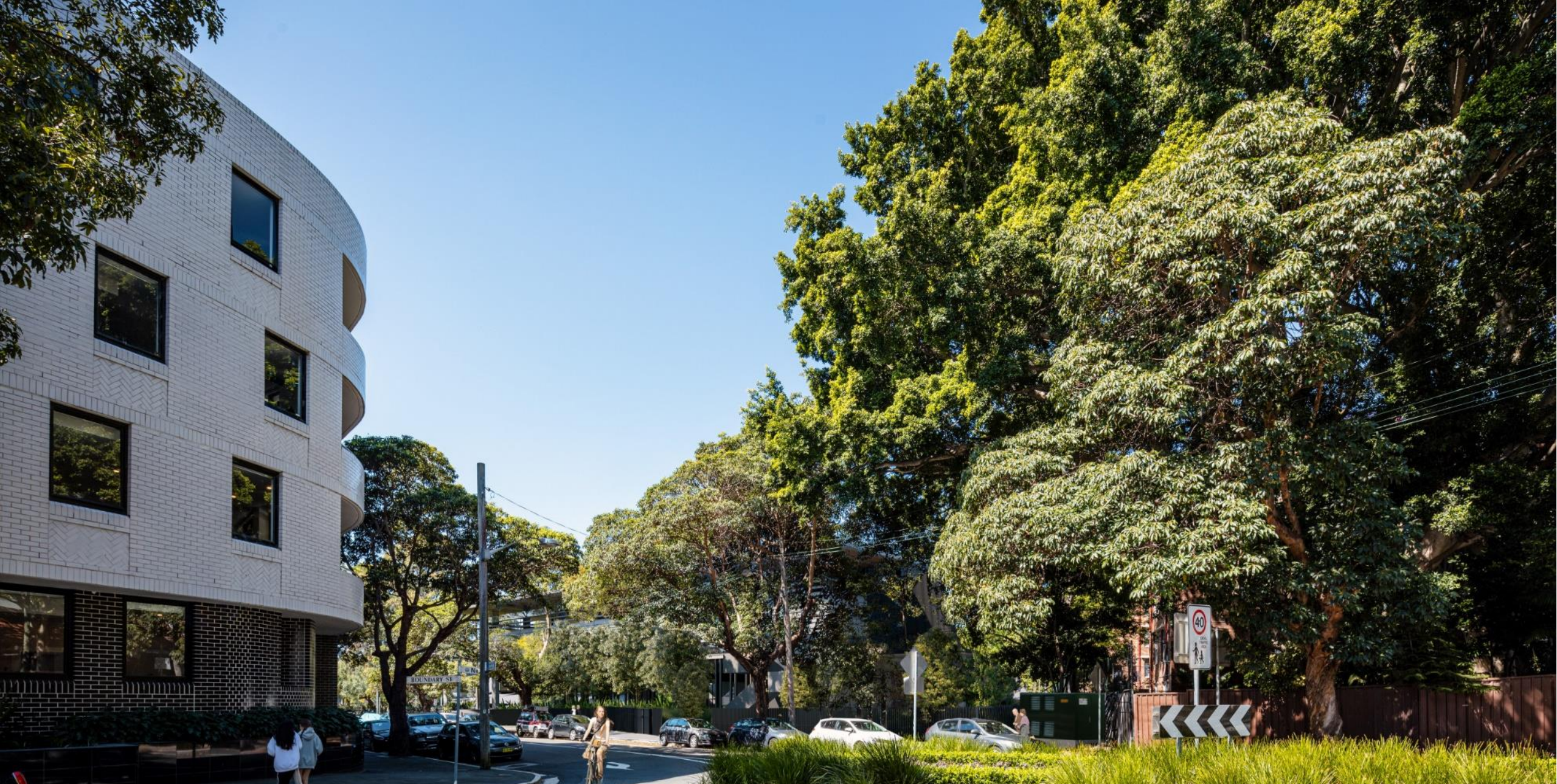
VIEW LOOKING NORTH EAST AT BOUNDARY STREET/NEILD AVENUE INTERSECTION
