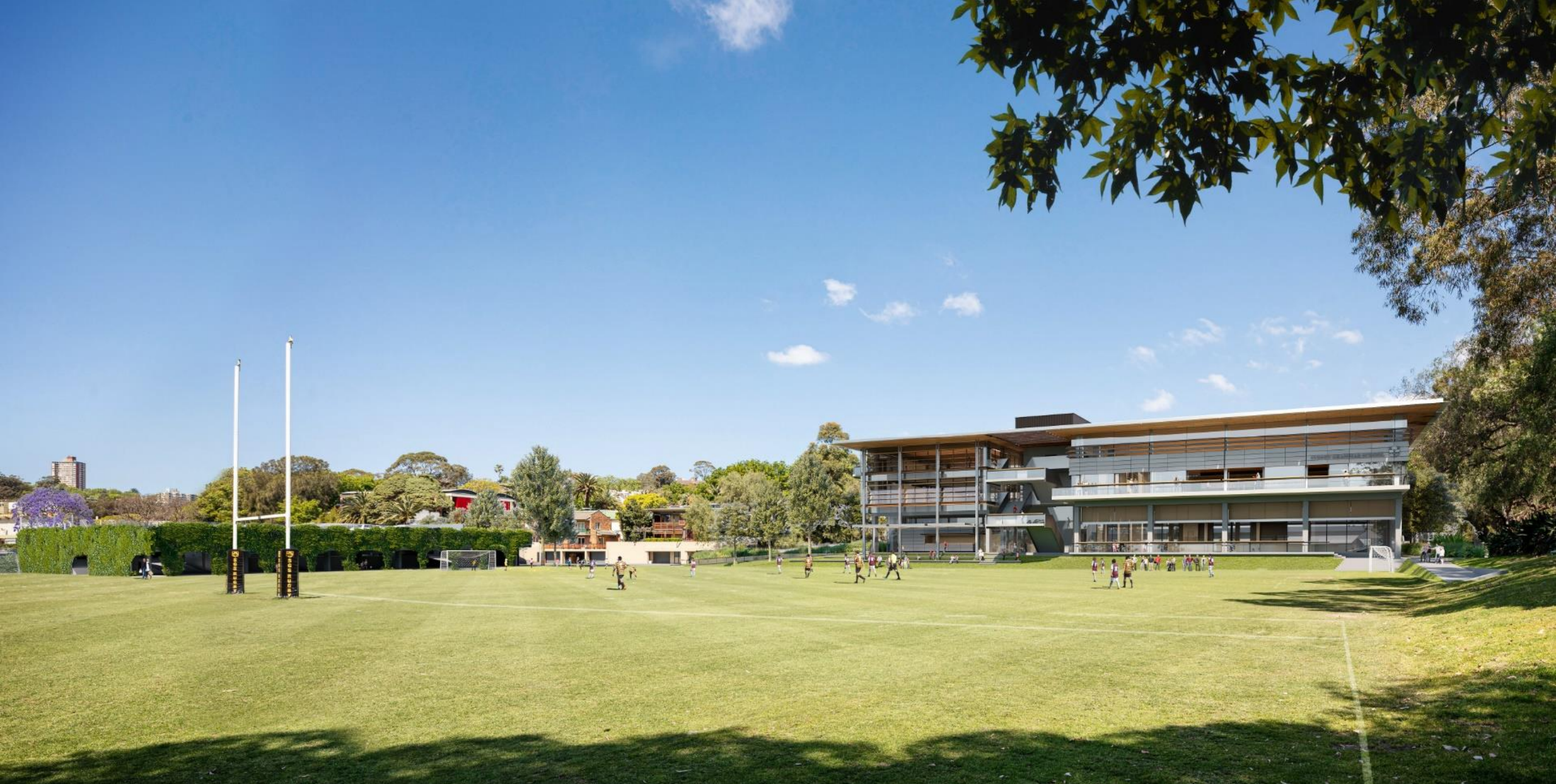
VIEW OF WEIGALL SPORTS COMPLEX LOOKING SOUTH FROM PLAYING FIELDS
