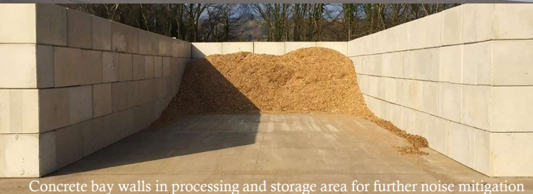
Concrete bay walls in processing and storage area for further noise mitigation
