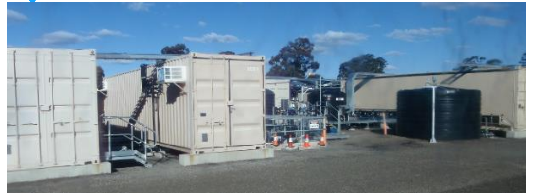
Modular water treatment system by Reverse Osmosis
