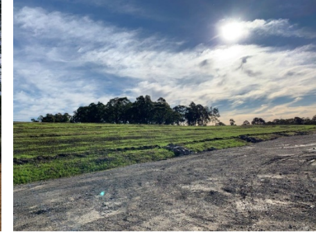
Macquarie Coal Closure Project (progress)
