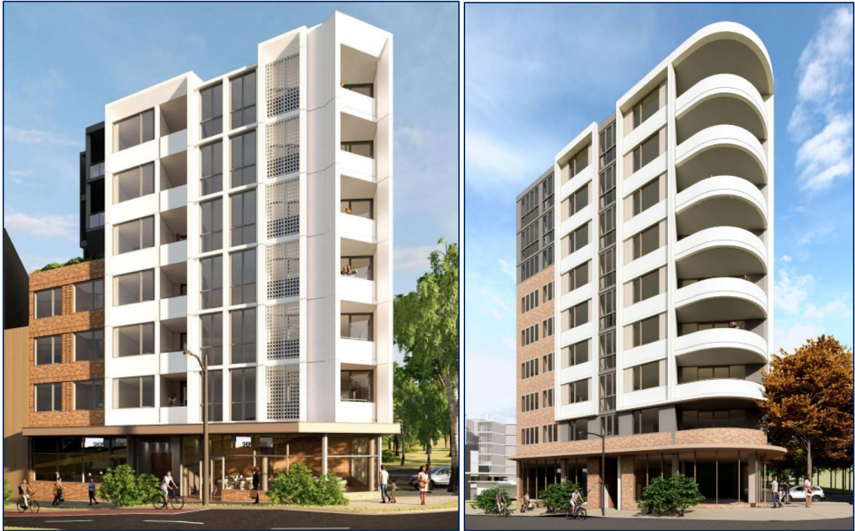
Figure 5 | Building B façade approved DA (left) and proposed (right) along Pittwater Road
