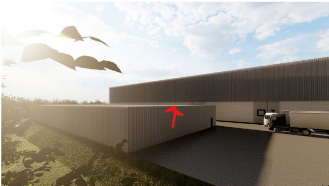
Western facade and waste water treatment building
