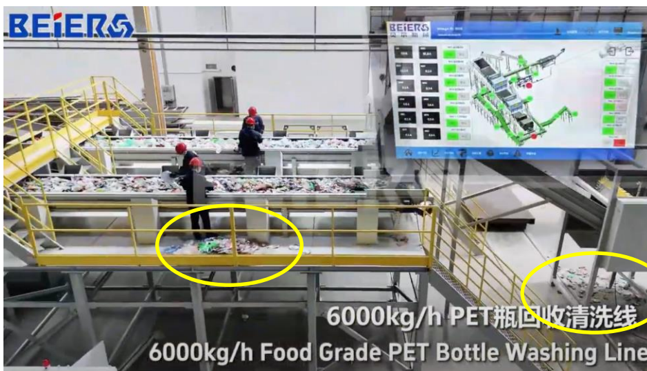
Figure B 2 - Contaminated and flammable waste spilt onto floor as circled.
