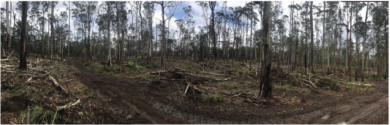
un-drained Snig-track at 5 degrees slope, draining in too head of mapped stream with no sediment control.
