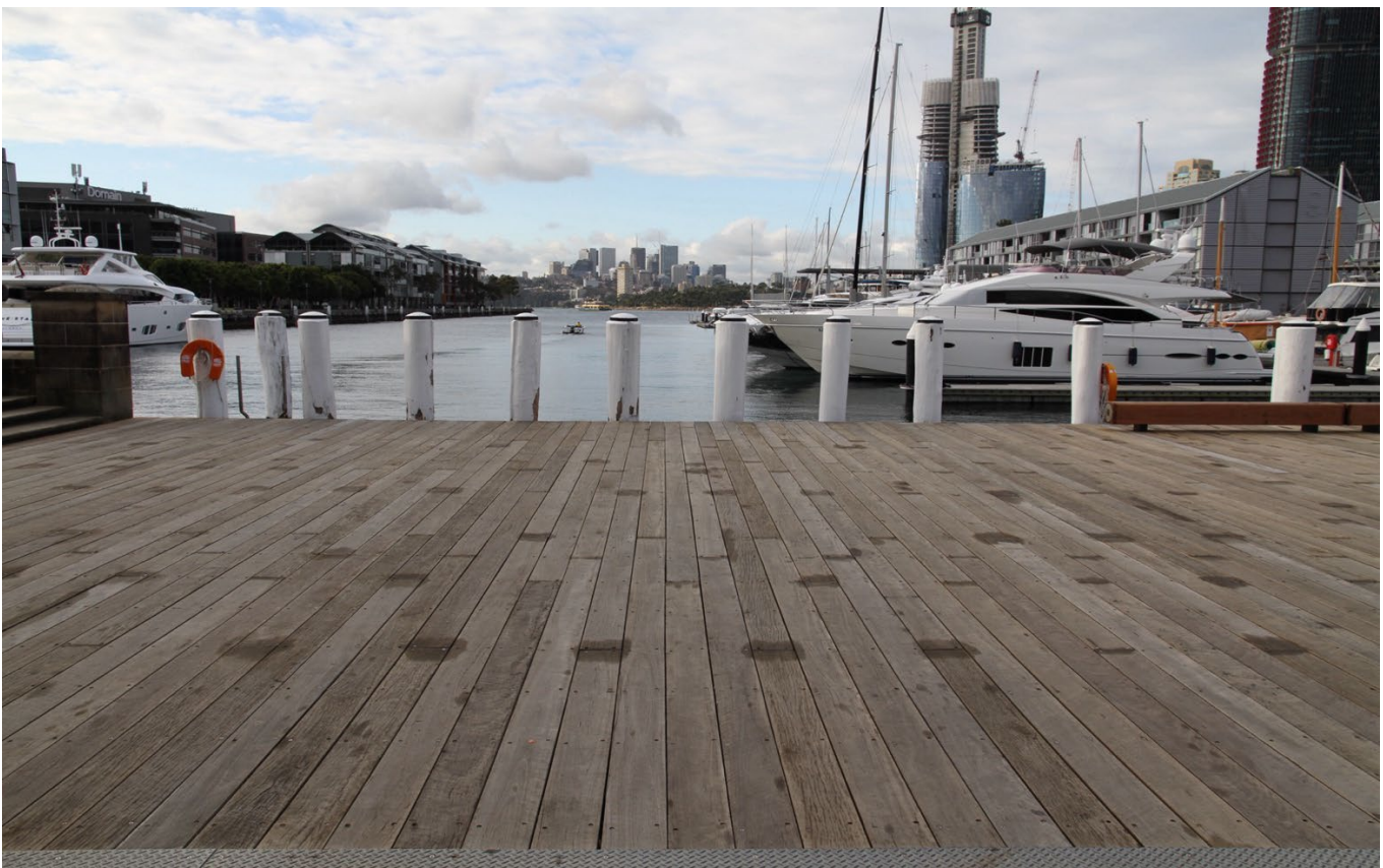
Wharf Decking for Infrastructure
