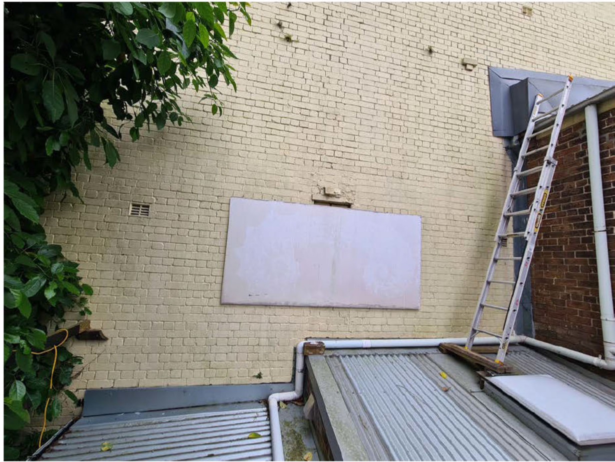
Figure 26: It is unclear from the proposed plans and elevations what height the proposed ground floor wall to the boundary is proposed to be. I would request that the height of the wall be sufficient to finish above my existing single storey kitchen and bathroom roof (as pictured above) in order to avoid a potential water ingress and maintenance issue of having a weird small section of lower roof between the two buildings along the boundary.
