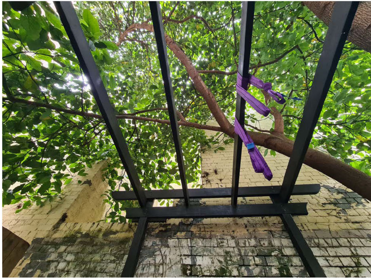
Figure 22: Photograph of the existing southern wall along the boundary between No. 6-8 Woodburn Street and No. 9 Woodburn Street. I request that this wall be retained to the boundary in this location and incorporated into the new construction of the proposed ground floor commercial space. If it is not possible to retain this wall, I request that the new wall be the same quality face brick as used elsewhere in the development.
