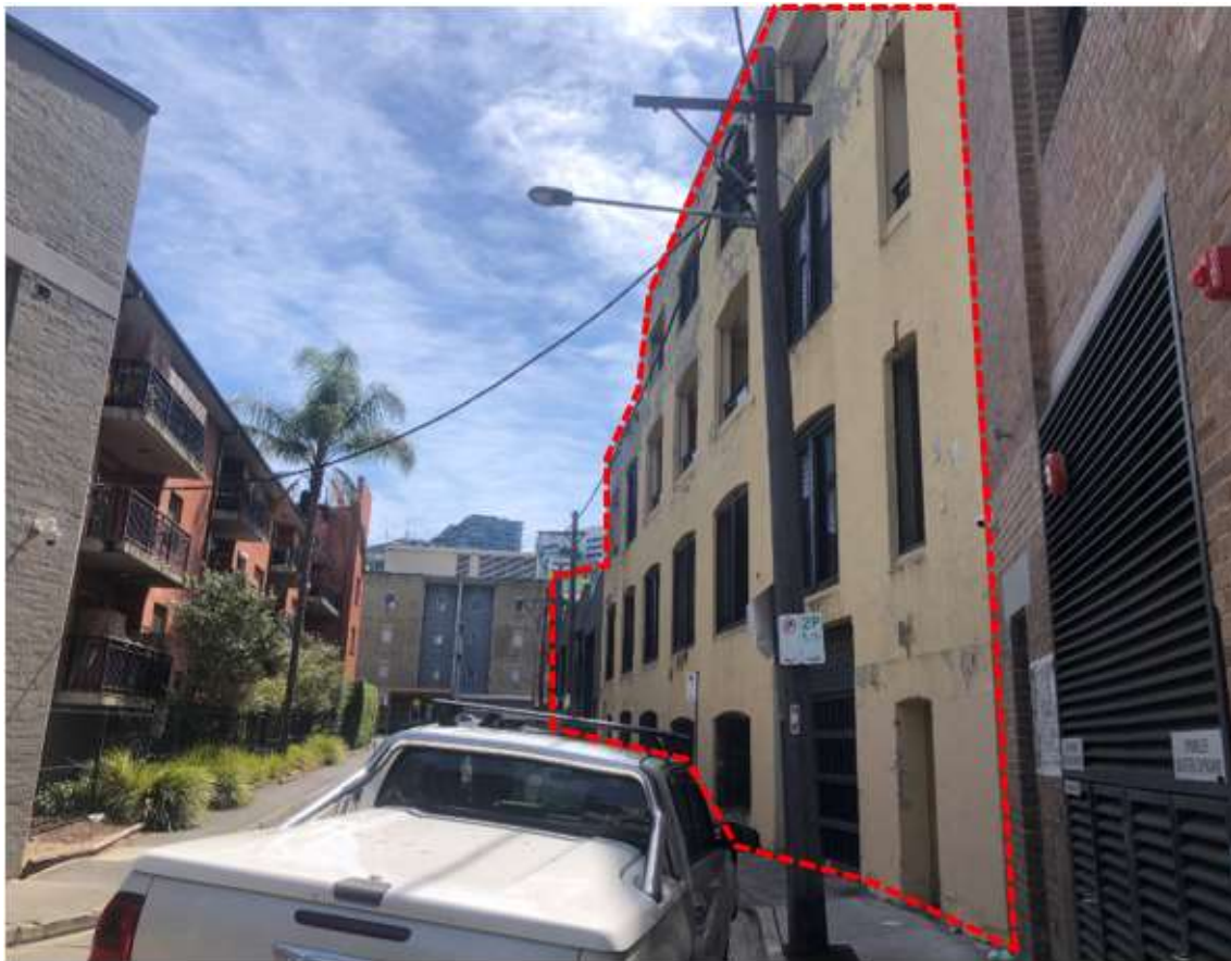
Figure 3 | View from Eveleigh Street looking north (Site in red)
