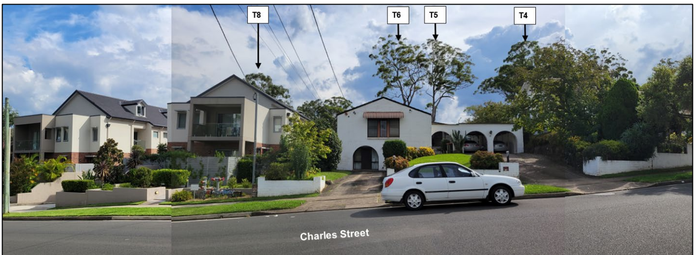
Figure 8 | View west towards low and medium density dwellings fronting Charles Street (Base source: Site visit 08 April 2024)
