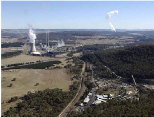
Springvale Colliery in foreground, Mt Wallerawang Power Station in middle ground and Mt Piper Power Station in background.
