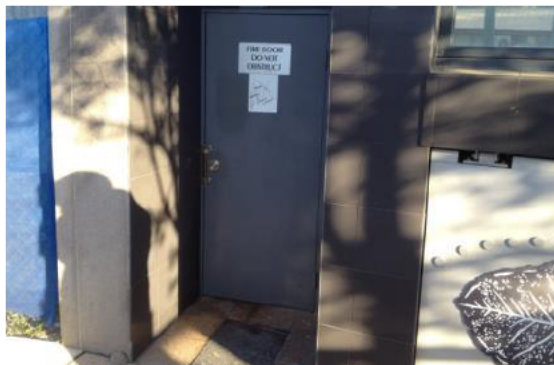
Figure 5: Fire Exit at Ground Level Example 2
