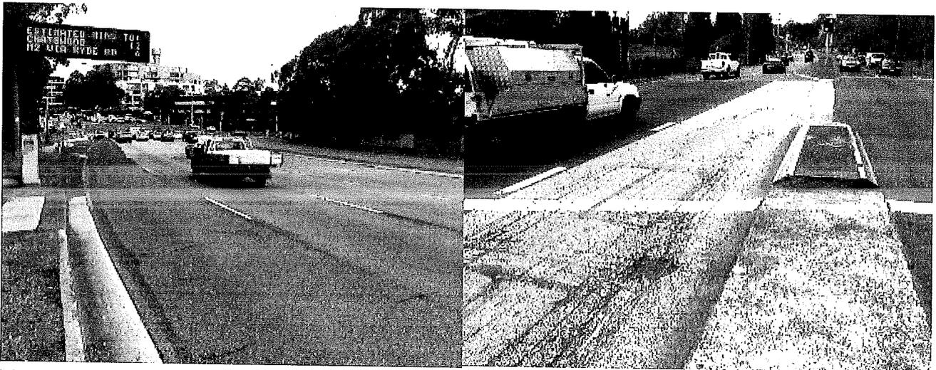
Photograph 16: Rhyolite intersection Pacific Hwy A1, Pymble in poor condition and a Rhyolite turning lane, Warringah Road Forestville in poor condition (24-6-2021).
