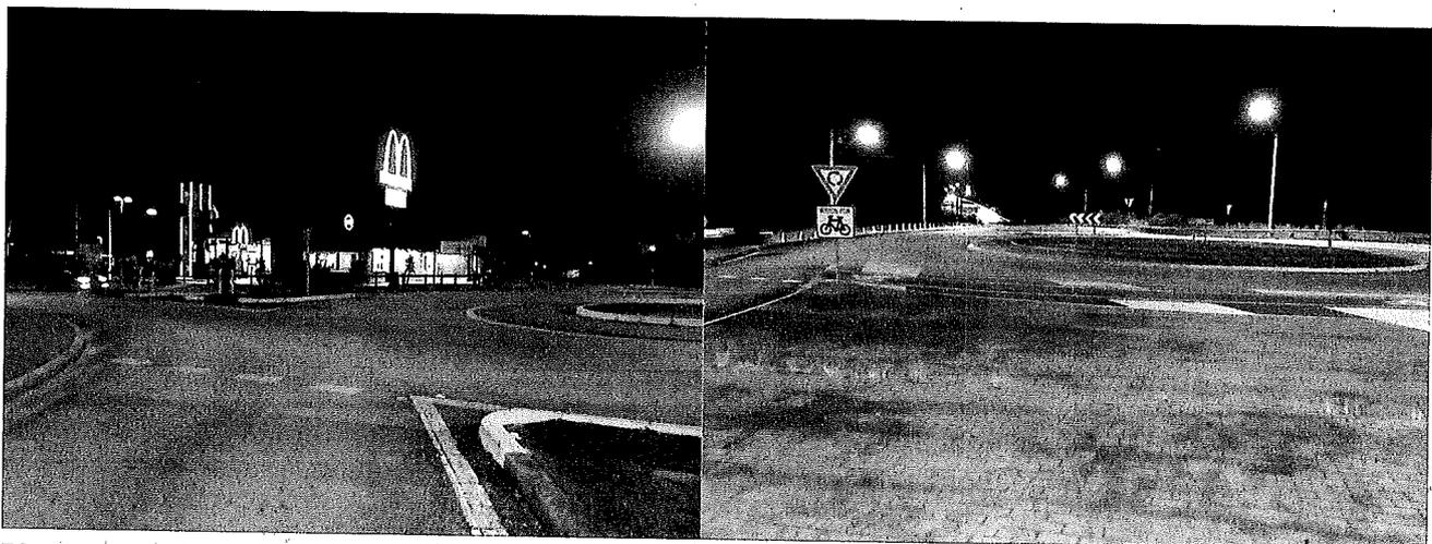
**Photograph 12:** Roundabout under lights Dora Street, Morisset, and Wangi Road, Rathmines on 24-6-2021, note the lighter materials improve the visibility of the road.
