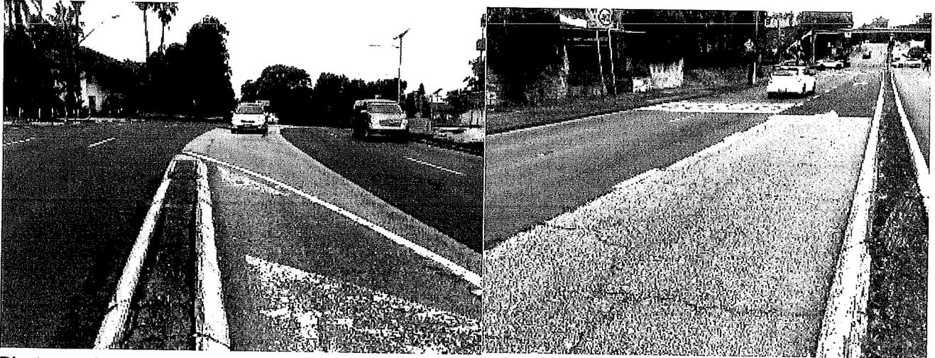
Photograph 15: Rhyolite turning lane Pacific Hwy A1, Wahroonga 24-6-2021 in poor condition.
