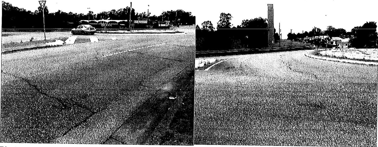
**Photograph 10:** Rhyolite roundabouts on Victoria Street and Northcote Street, Kurri Kurri in poor or deteriorating conditions on 16-3-2021.
