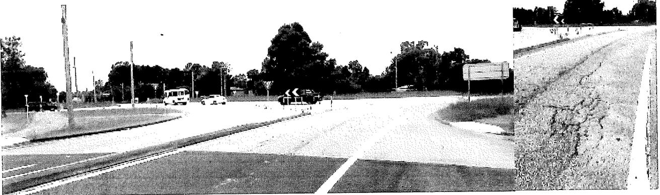
Photograph 7: Rhyolite roundabout at Salt Ash 20-1-2021 in poor condition.
