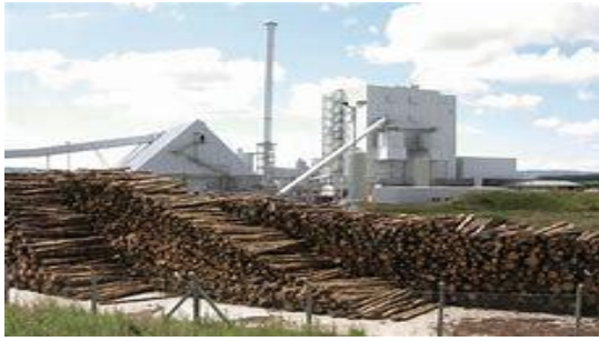
Biomass power plant
