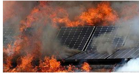
PV solar panel fires create toxic smoke
