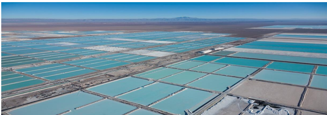
Extraction of lithium pumped from underground salar (salt flat) brine deposits into evaporation ponds
