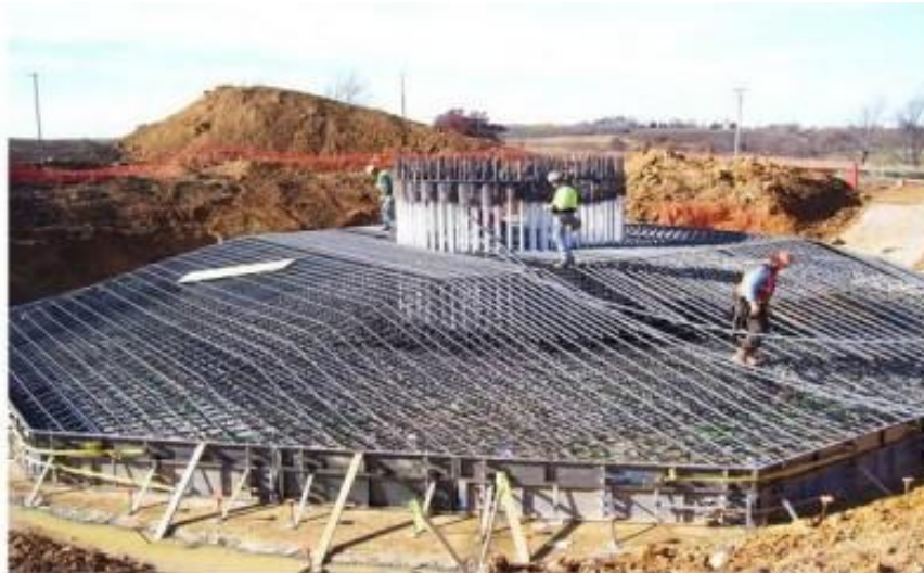
A single 1MW wind turbine concrete base under construction
