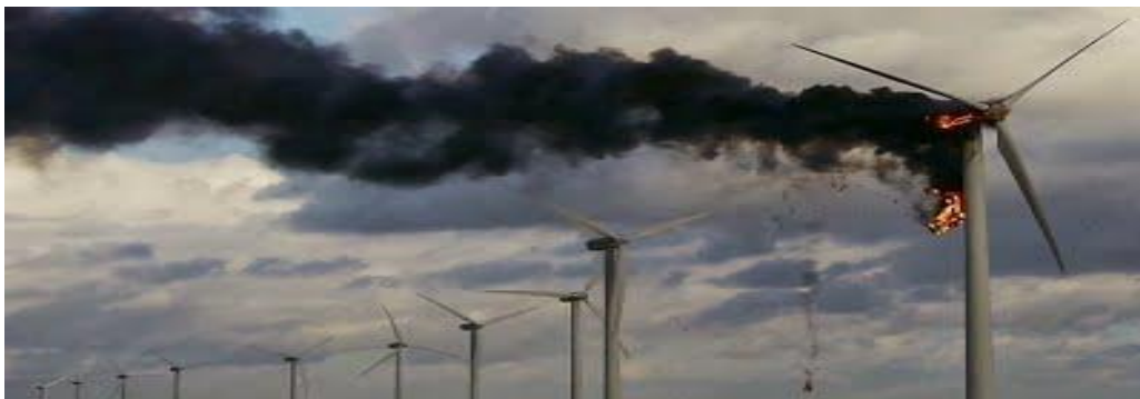
Wind turbine on fire
