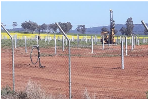
Land cleared. cables laid. pile-driven uprights in place
