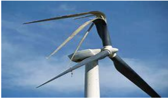
Lightning strike shuts down wind turbine
