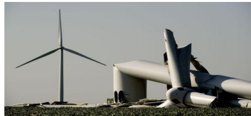
Wind turbine collapse impacts output
