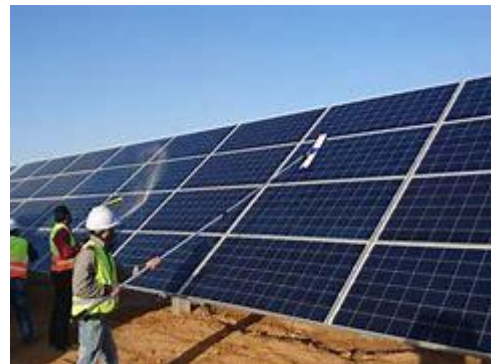
Cleaning PV solar panels
