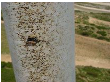
The build up of dead insects reduces the output. Insects attract birds. Blade tip speed can exceed 280kmph
