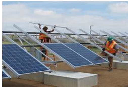
Crew of two install cross-members and panels
