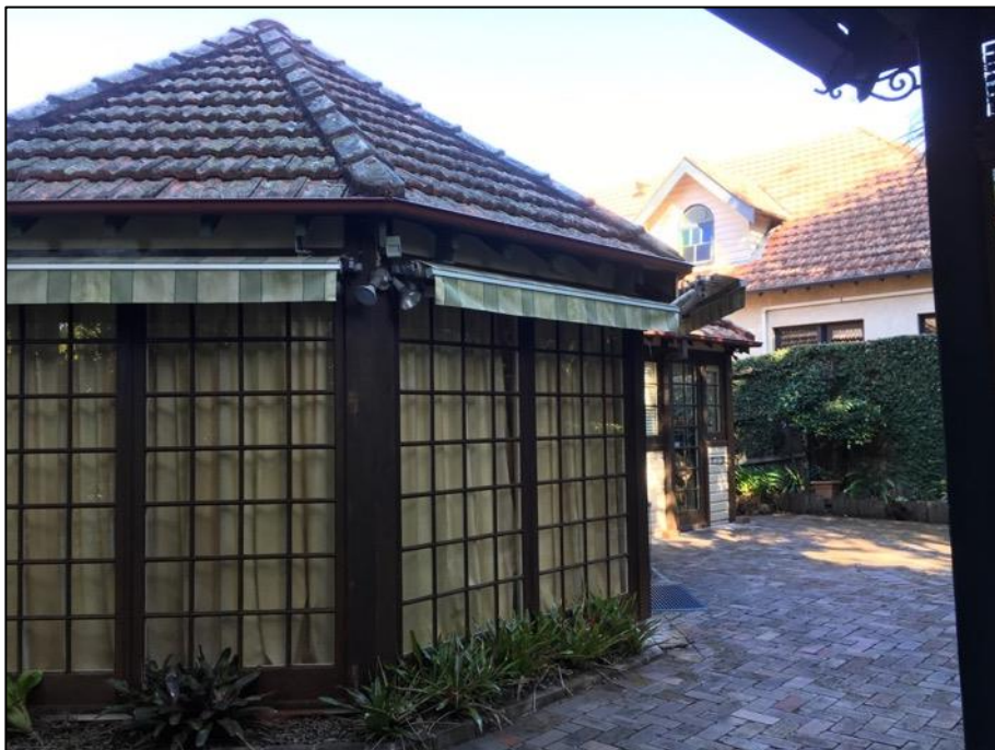
Figure 6: Rear garden and rear elevation to No. 115 Holt Avenue.
