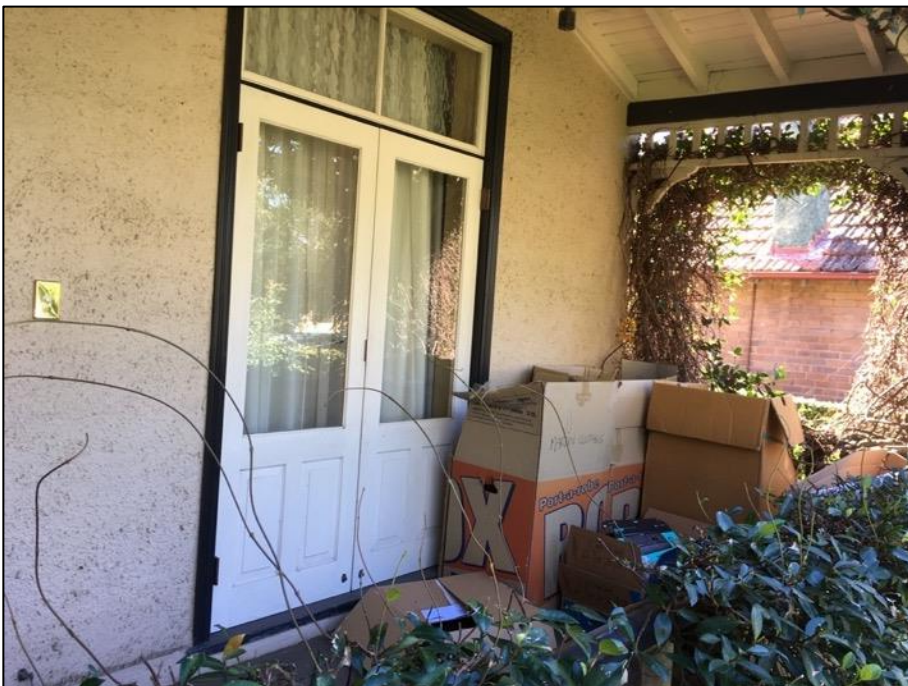
Figure 23: Close-up of front elevation showing French door and verandah.
