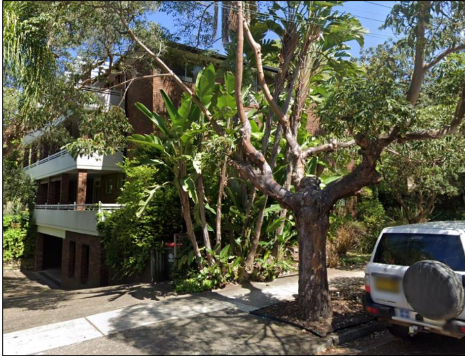
Figure 51: No. 132 Spencer Road to the northwest of the site.
