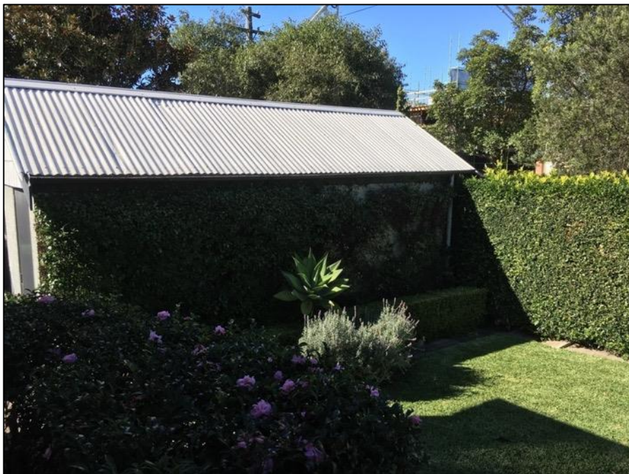
Figure 35: Garage at the front of site.
