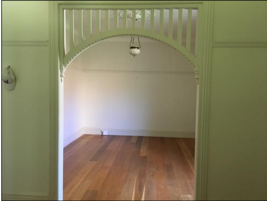
Figure 42: The front two formal rooms separated by an arched opening with a timber architrave.
