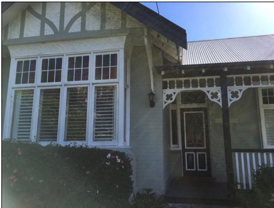
Figure 38: Close-up of front elevation showing bay window and verandah.
