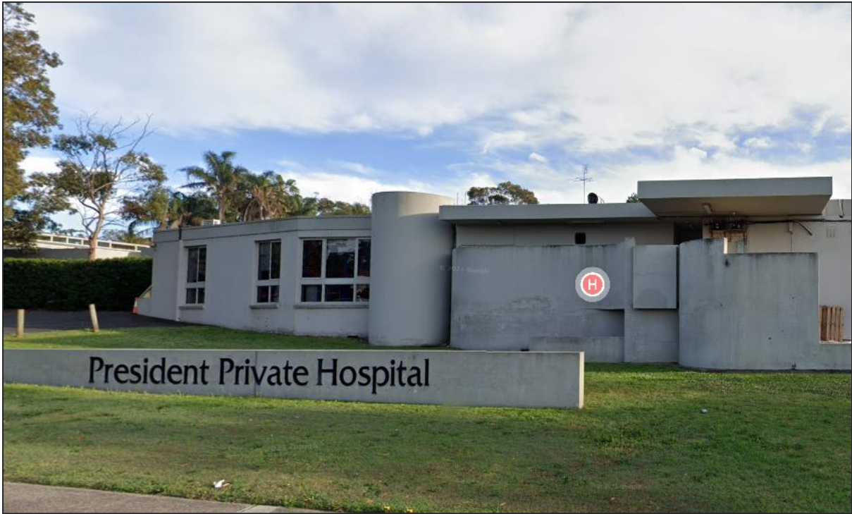
Figure 4 | Existing hospital building (Source: Neamap 2022)
