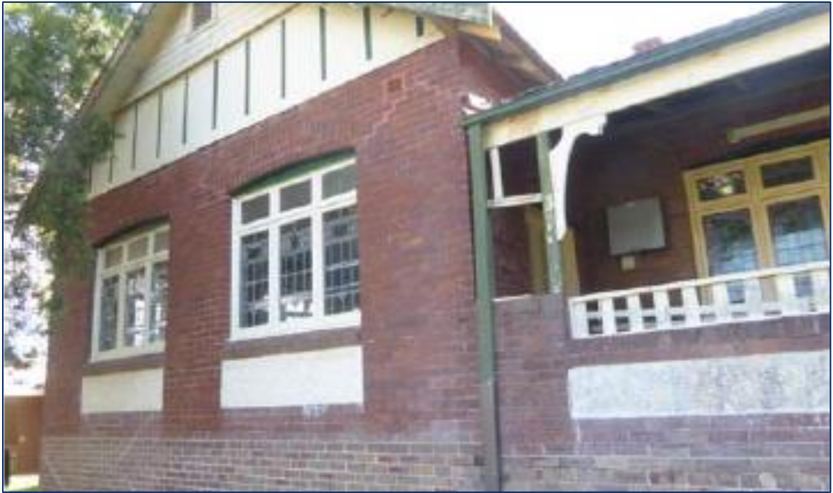
Figure 29 | Ballroom brickwork addition (Source: GBA Heritage 2020)
