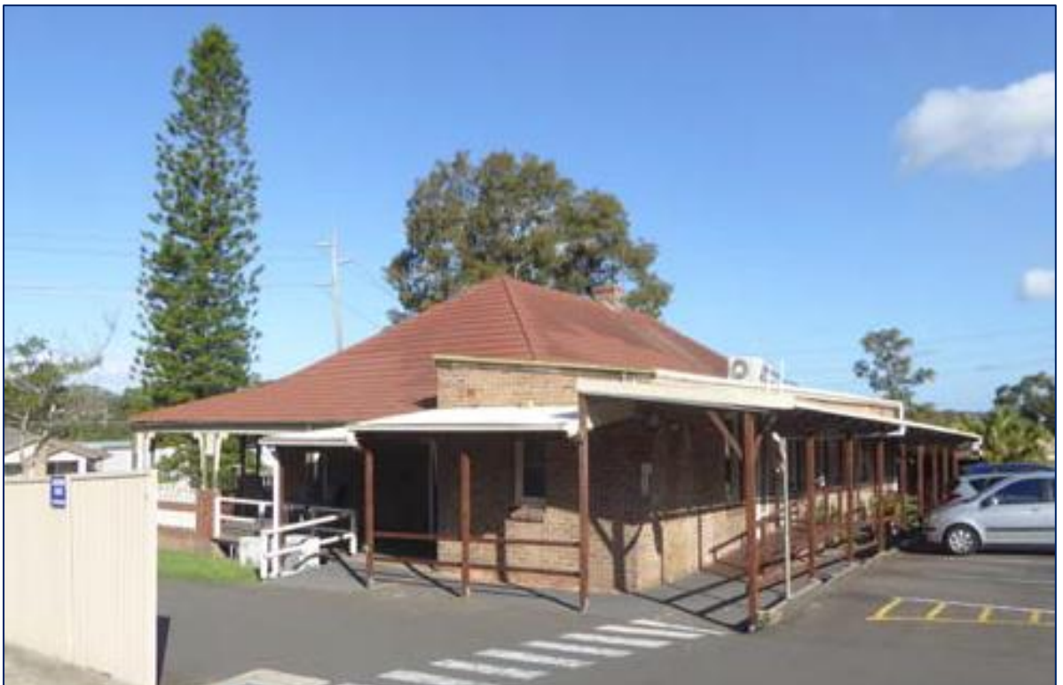
Figure 30 | Rear view (Source: GBA Heritage 2020)
