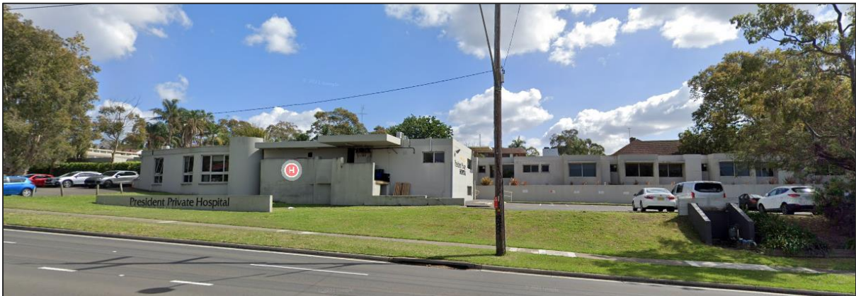
Figure 5 | Existing hospital building (Source: Neamap 2022)
