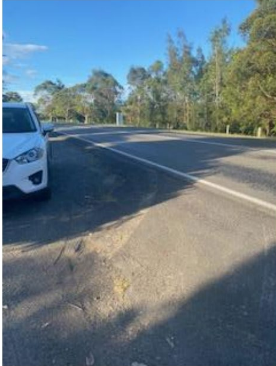
View facing North from edge of driveway
