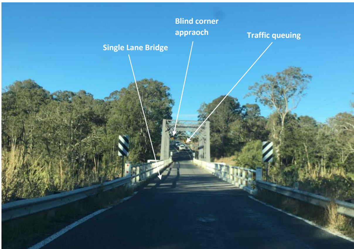
Gostwyck Bridge, single lane timber bridge, Dungog Road
