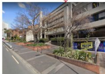
Figure 18. Aerial image and street view of the south side of New South Head Road (Source: Google Maps 2020 modified by Council staff)
