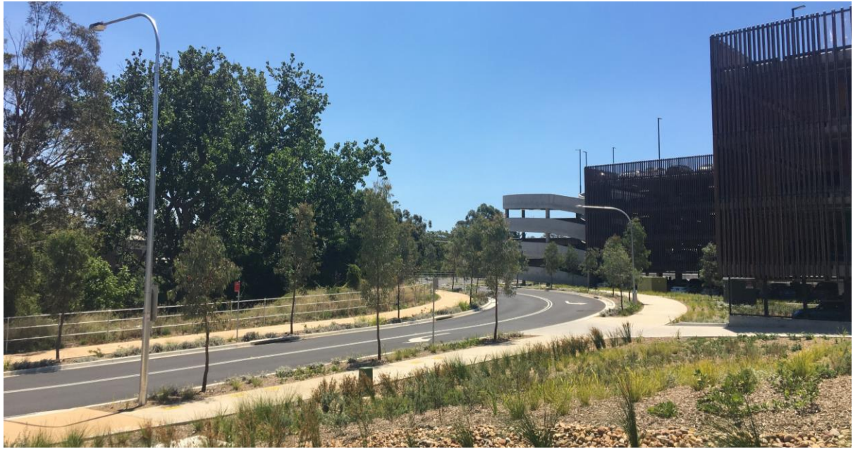
Figure 6 | Interface between Cattai Creek and commuter carpark viewed from Carrington Road
