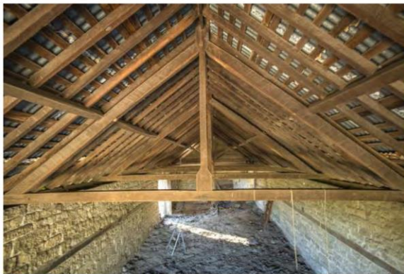
Roof structure of the Barn.
