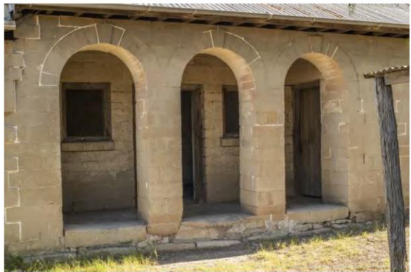
Arched columns on east elevation of Stables
