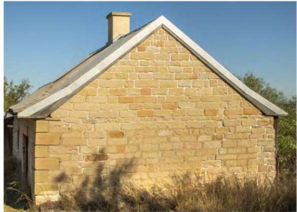
North elevation of the Barn showing the bellcast eaves
