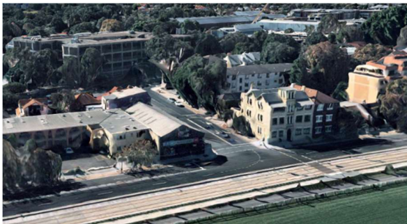
3D image 1: Mar 19 – NE view of Alison Rd
