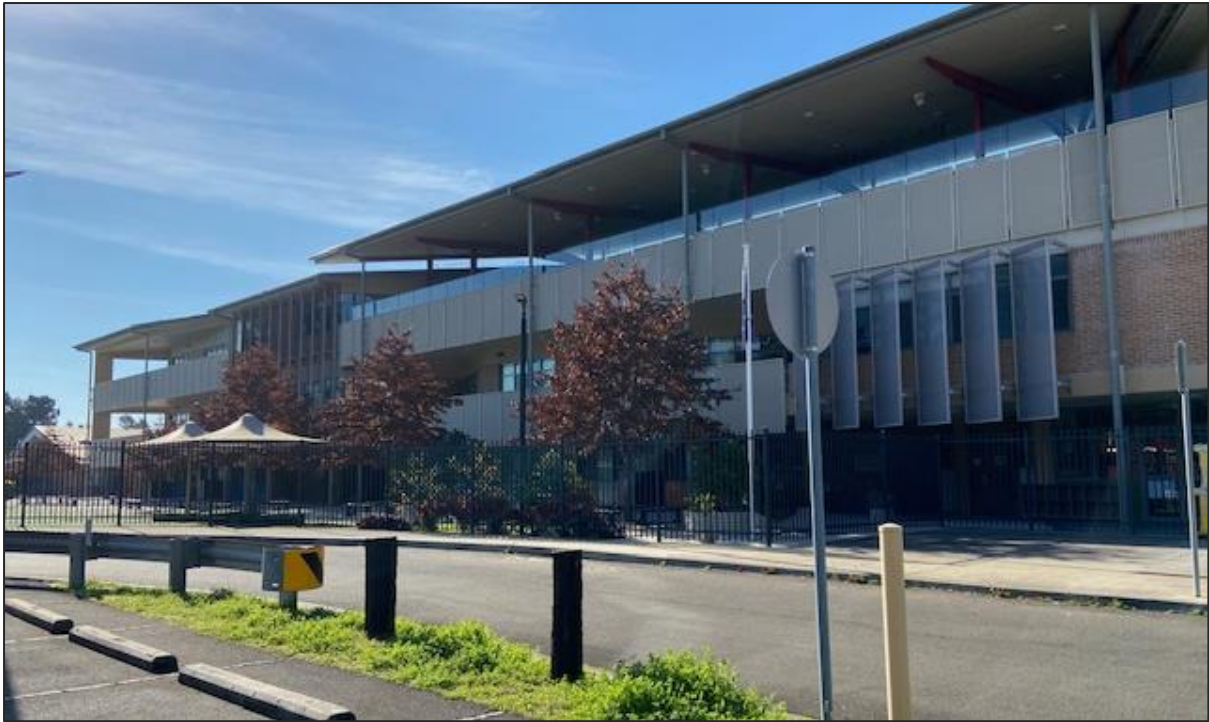
Figure 7 | Project site – looking east towards existing primary school building (Source: DPIE 2020)
