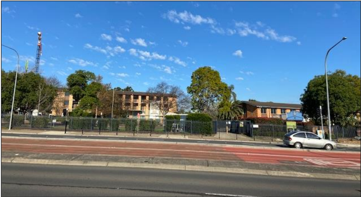
Figure 4 | WCC site from Darcy Road – looking south-west (Source: DPIE 2020)
