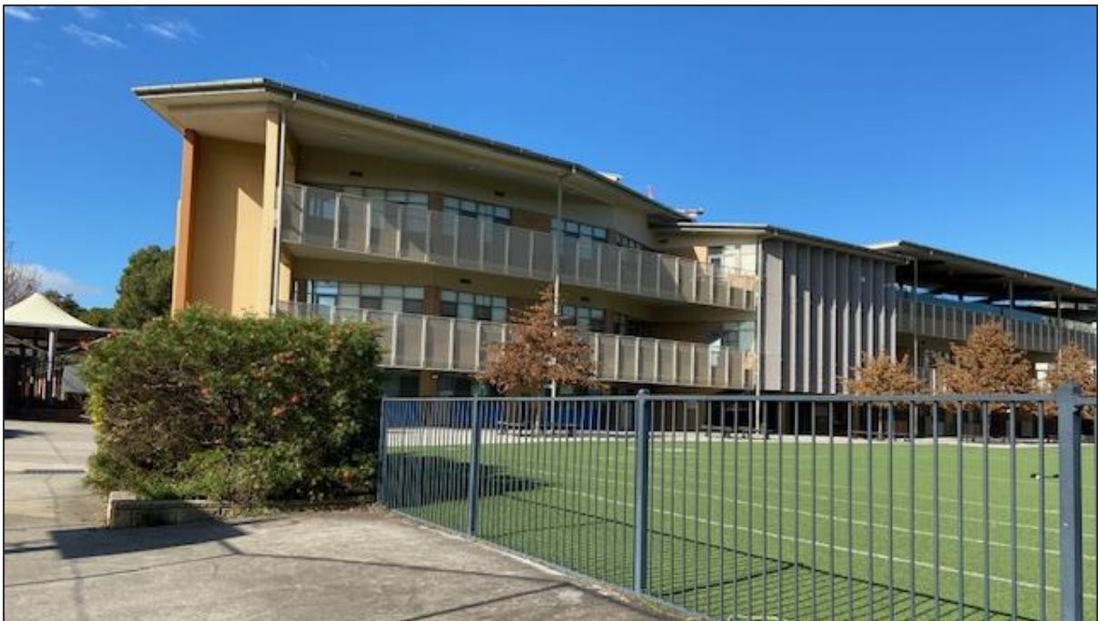
Figure 8 | Project site – looking east towards existing primary school building (Source: DPIE 2020)
