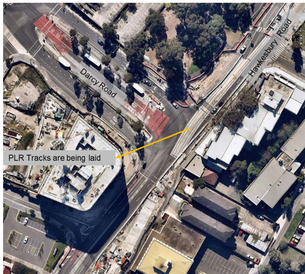
Figure 4.2: Darcy Road / Hawkesbury Road PLR Construction Work
