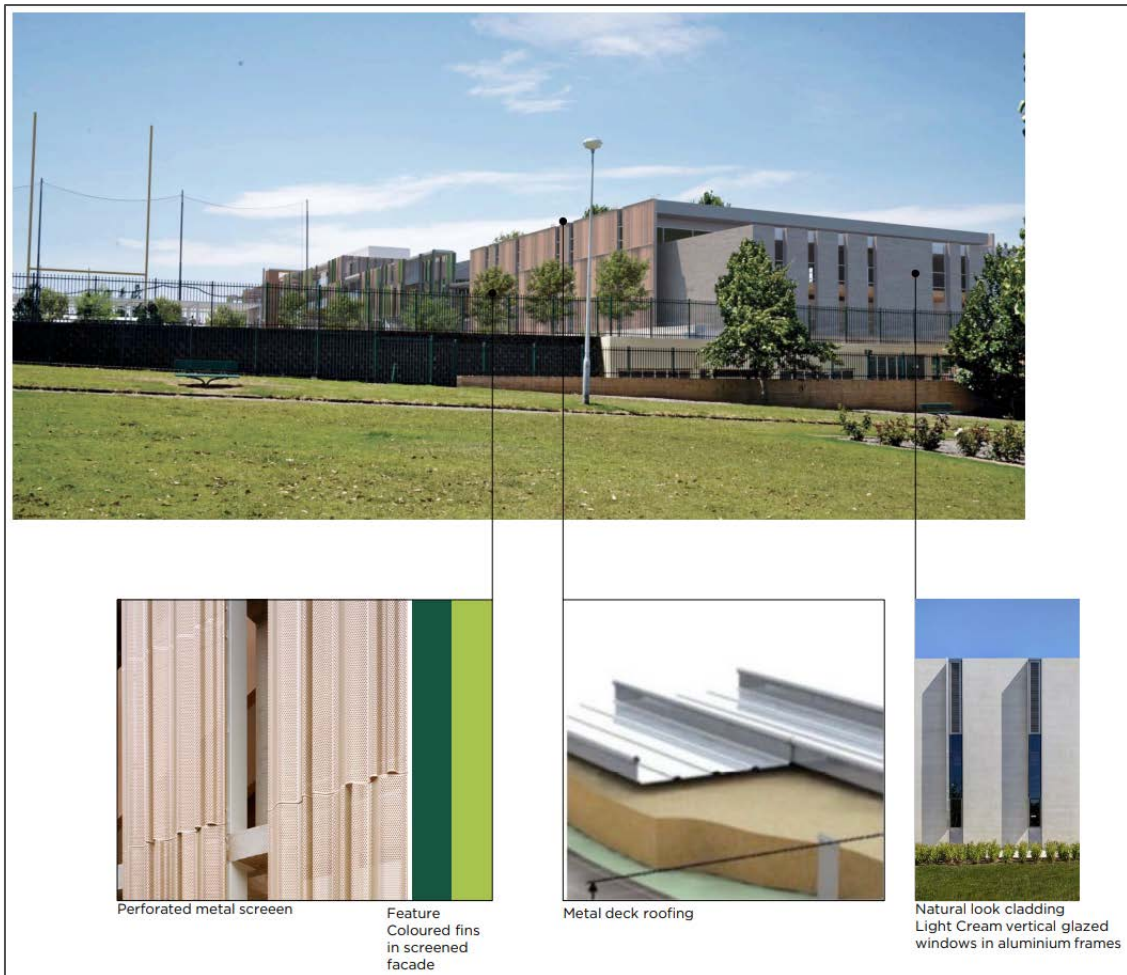
Figure 34 | Southern view of the Multi-purpose pavilion showing the scale and proposed façade treatments (Source: Applicant's SRtS 2021)
