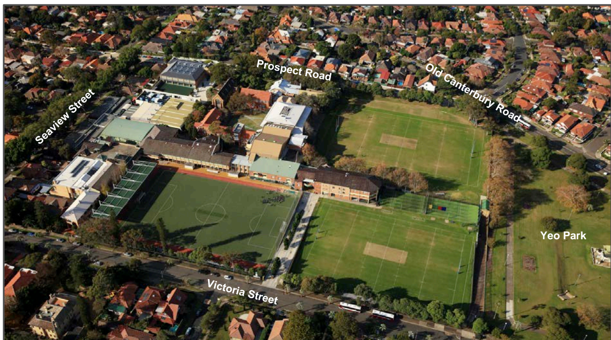
Figure 5 | Aerial view of site and surrounds (Source: Applicant's EIS 2020)
