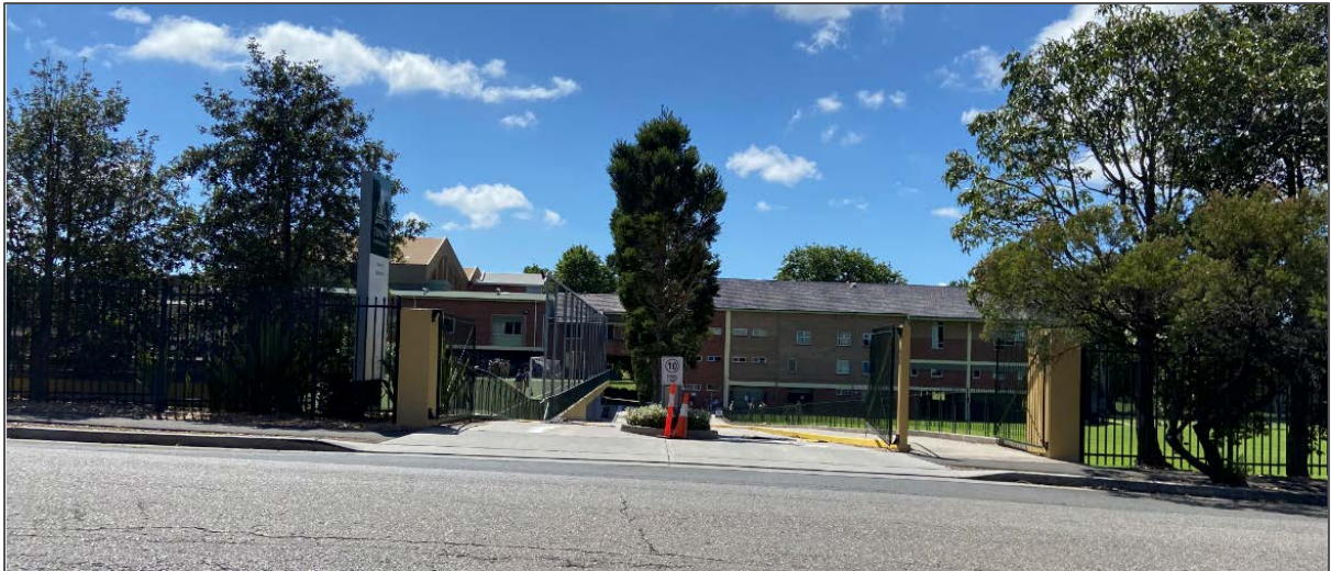
Figure 6 | Vehicle entrance to underground car park on Victoria Street (Source: DPIE 2020)
