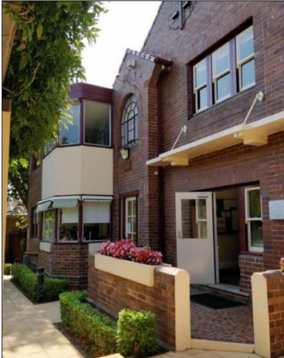
Student Services Building
