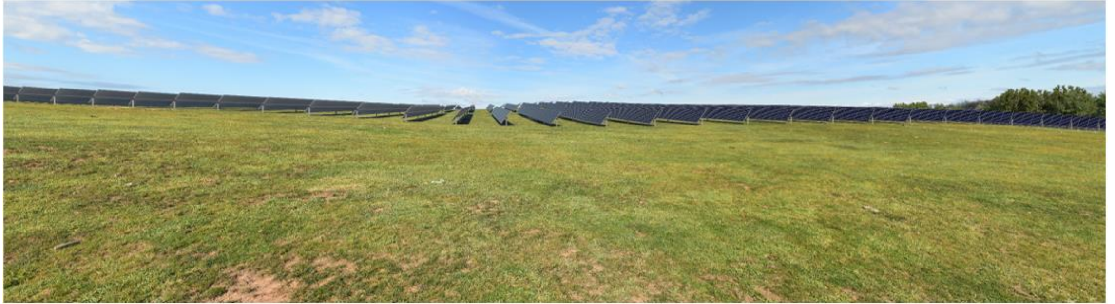
Photomontage looking south towards the site from Residence R35 with a 50 m setback without visual mitigation
