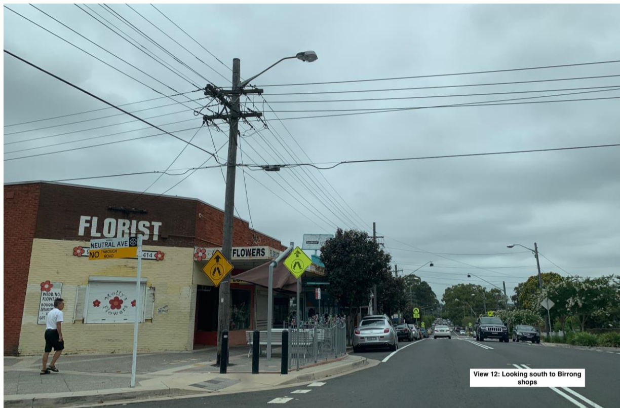
Figure 13 – View 12 looking south to Birrong shops
