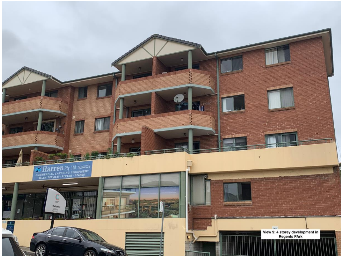
Figure 10 – View 9 of a 4-storey development in Regents Park
