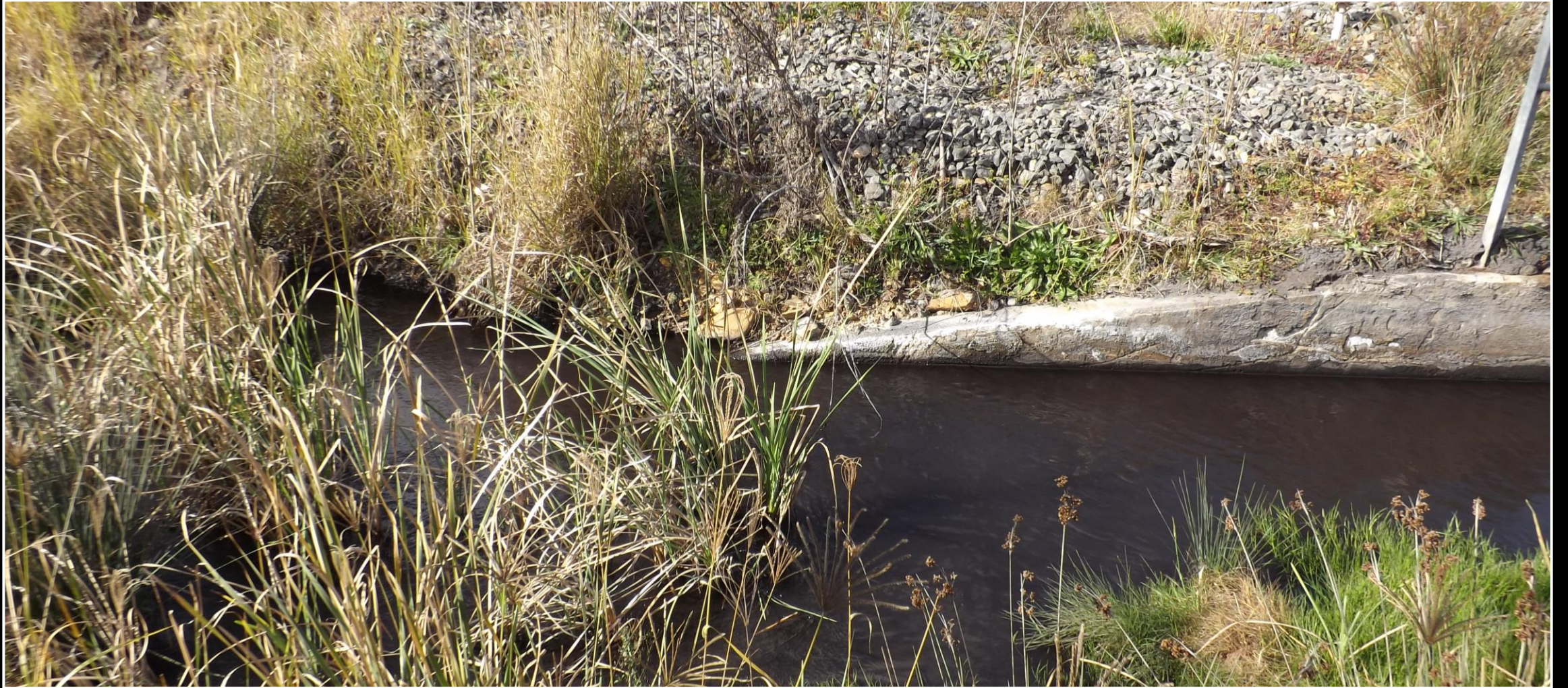
SIMEC wastewater discharge – turbidity 23 rd Jul 2020
