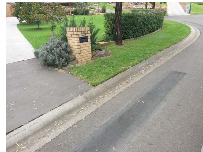
Stonequarry Creek Road - Image 3(b)
