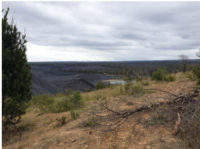
Refuse Emplacement Area – Image 9(c)
