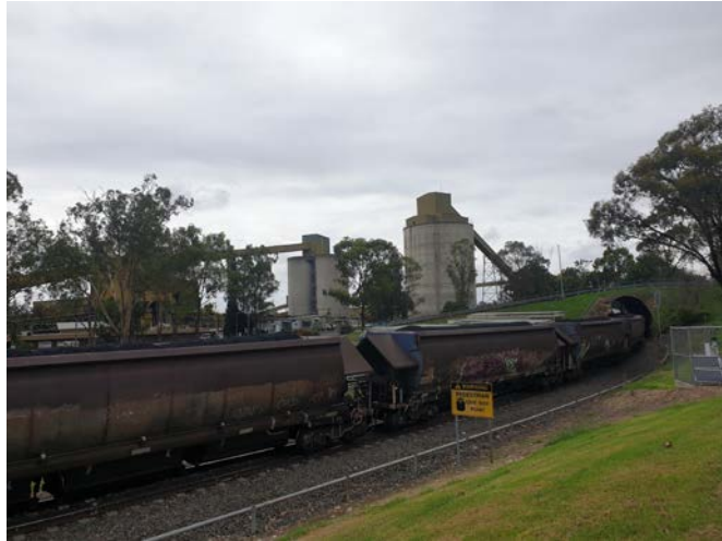
Tahmoor Coal Pit Top – Image 1(a)
