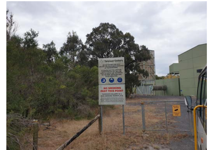
Existing Ventilation Shaft – Image 10(a)
