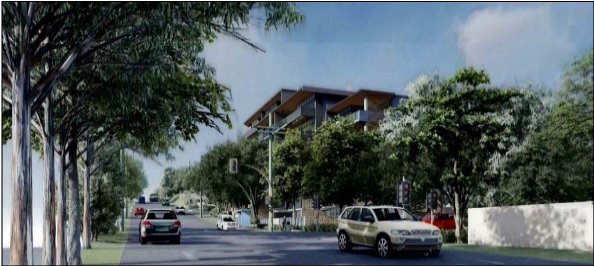
Figure 12 | Illustrative perspective of the development along River Road from the west (Source: RtS)
