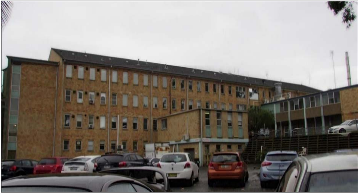
Figure 5 | Existing five storey hospital building (Source: EIS)
