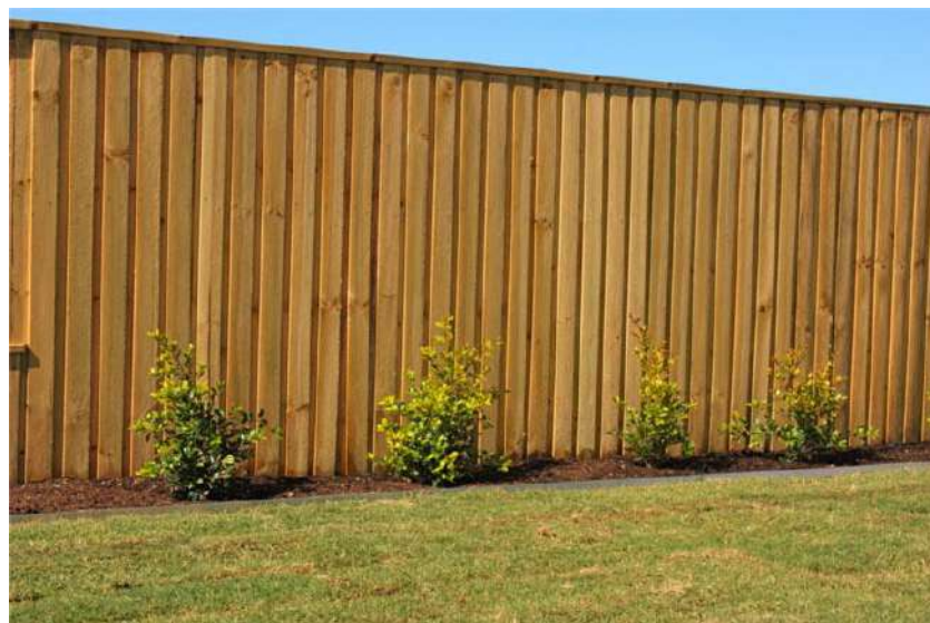
Figure 3-2 – Capped and lapped fence. Source: fencescape.com.au
