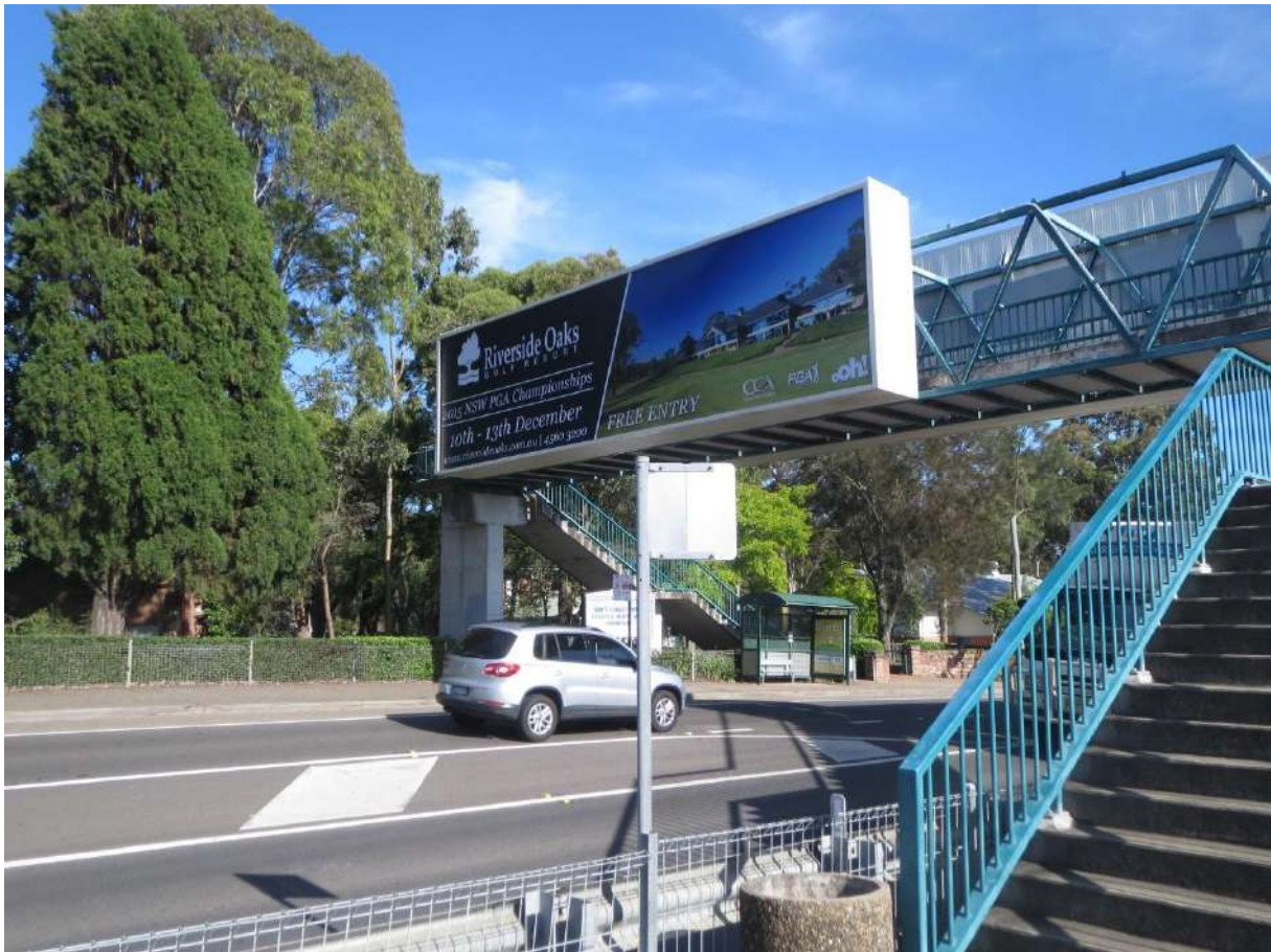
Figure 3 Pedestrian over pass
