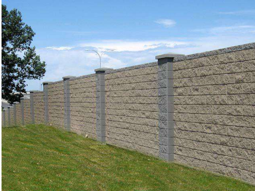
Figure 3-3 – Block wall. Source: arizonafencebuilders.com
