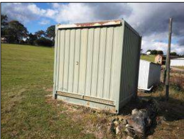
Photograph 21 – Chemical storage shed situated adjacent to the dam
