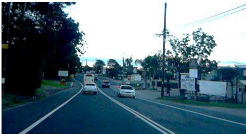
Figure 11 New Line Road south of Old Northern Road
