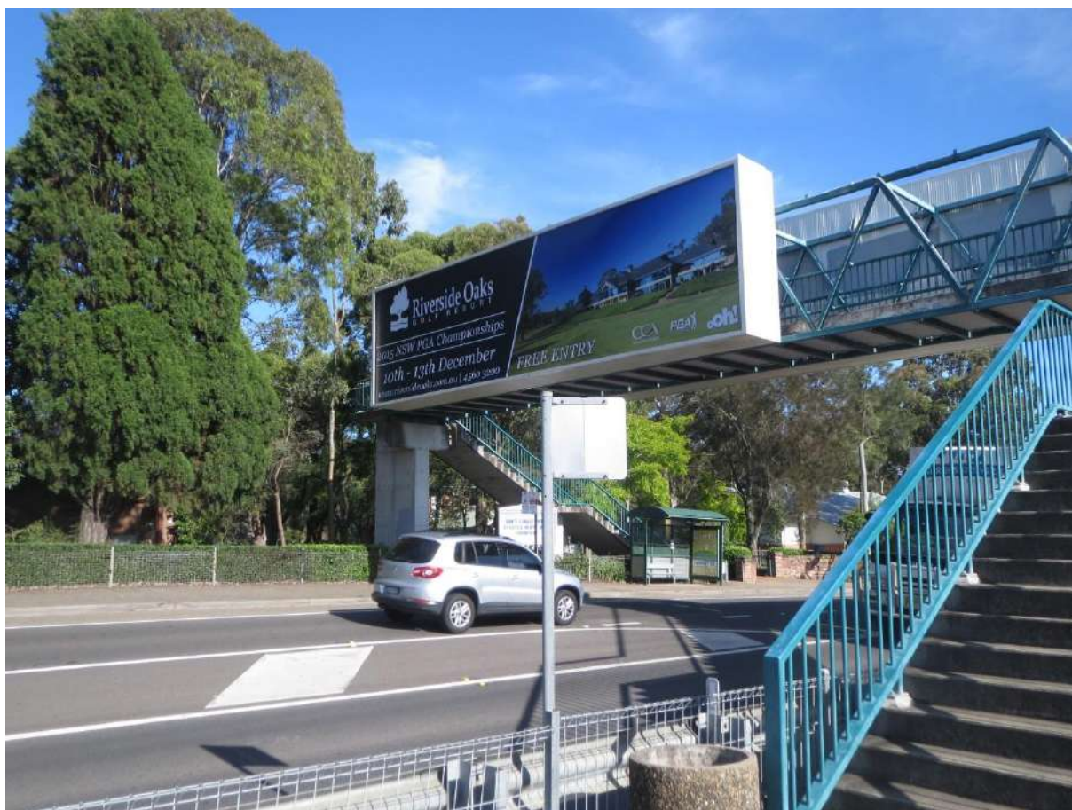
Figure 3 Pedestrian over pass
