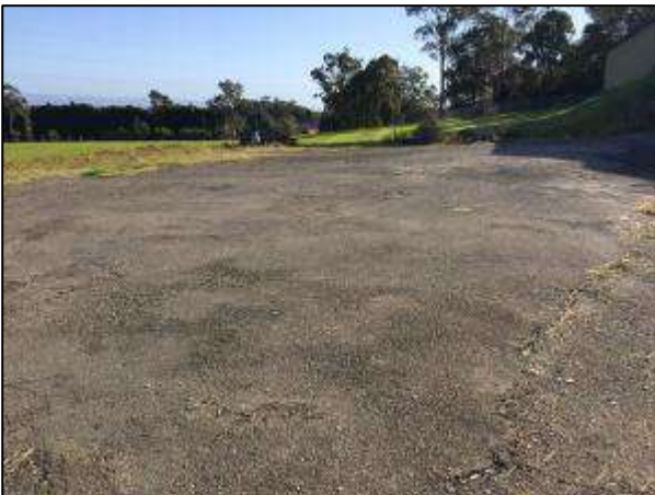
Photograph 9 – eastern carpark covered with asphalt
