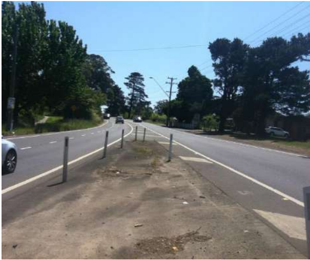
PICTURE 1 – THE OLD NORTHERN ROAD VIEW NORTH
