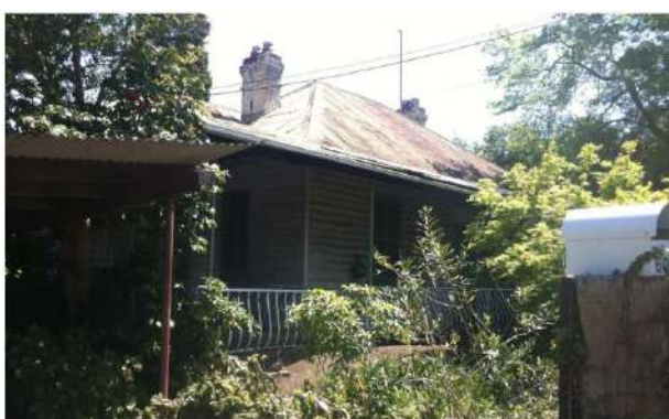
Picture 5 – Item 85: 600A Old Northern Road
