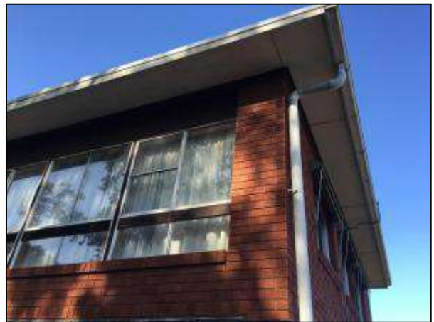
Photograph 17 – Residential house present, 1980s style construction
