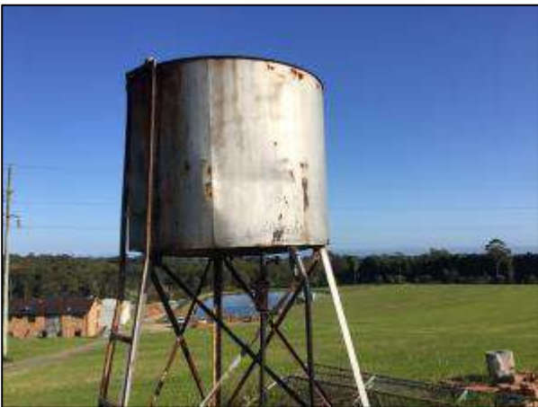
Photograph 8 – Above ground Storage Tank (AST).
