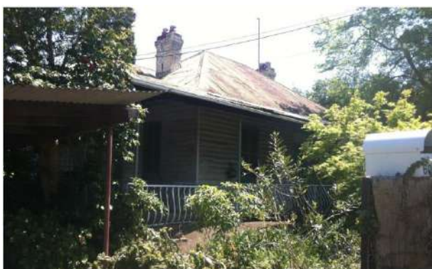
Picture 5 – Item 85: 600A Old Northern Road
