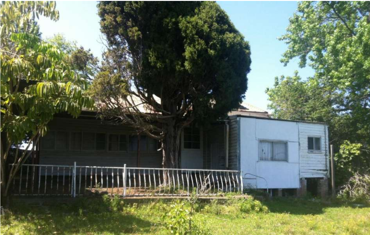
FIGURE 4 – REAR OF LISTED HOUSE 600A OLD NORTHERN ROAD.
