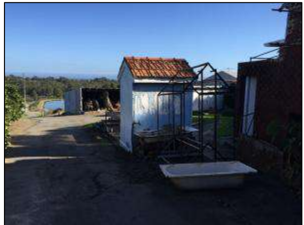
Photograph 18 – Asbestos cement shed present on southern exterior of residential building
