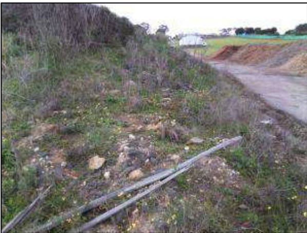
Photograph 26 – Southern dam wall and driveway
