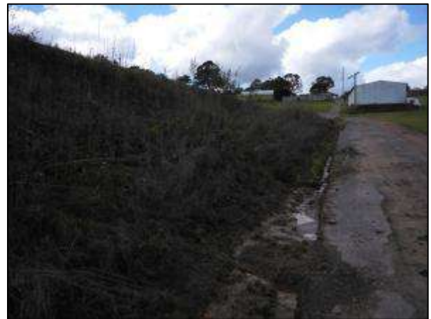
Photograph 29 – Southern dam wall facing east
