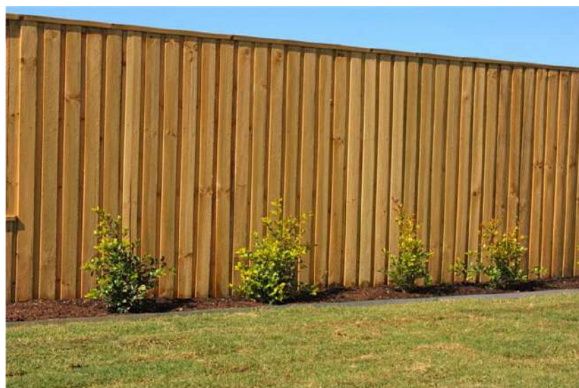
Figure 3-2 – Capped and lapped fence. Source: fencescape.com.au
