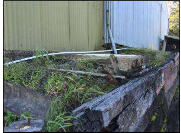
Photograph 10 – cement slab present adjacent to southern exterior of shed 1, potential previous location of tank
