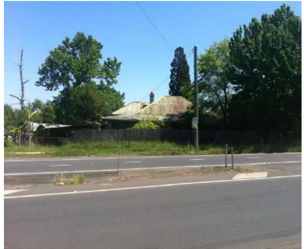
PICTURE 2 – LISTED HOUSE 600A OLD NORTHERN ROAD
