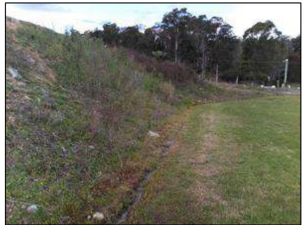
Photograph 23 – Western dam wall
