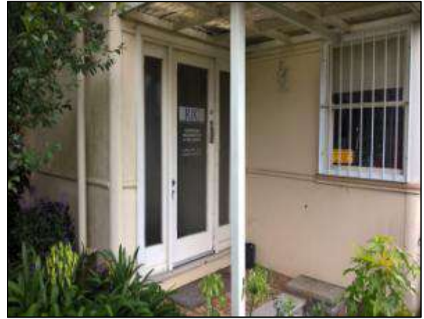
Photograph 4 – Front door to subject property
