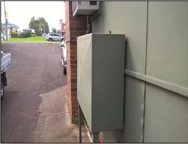
Photograph 7 – Approximately 150 L Caltex AST on the northern house exterior (facing south)
