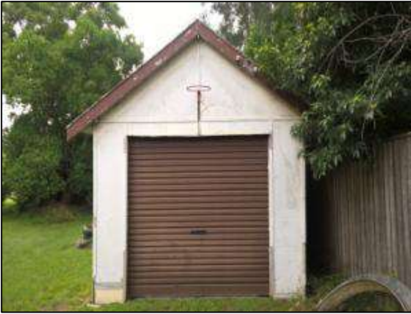
Photograph 7 – Garage constructed of presumed asbestos cement sheeting.
