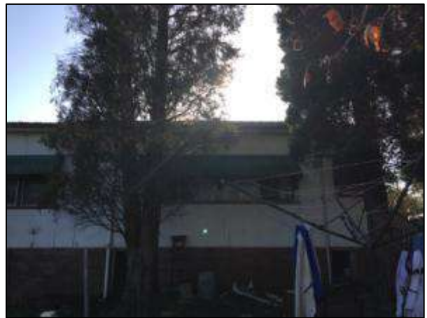
Photograph 11 – Exterior of house with asbestos sheeting
