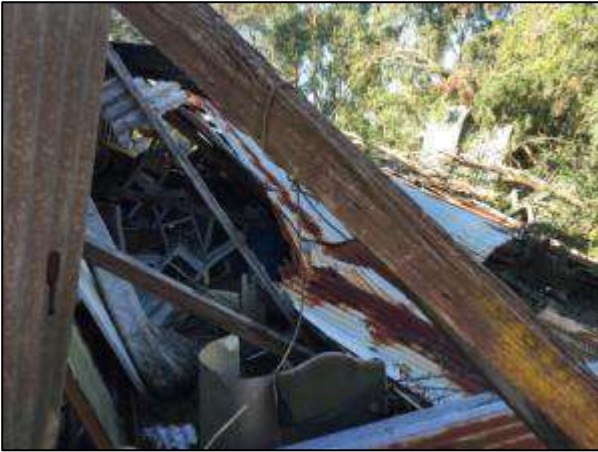
Photograph 7 – Demolished shed with corrugated iron
