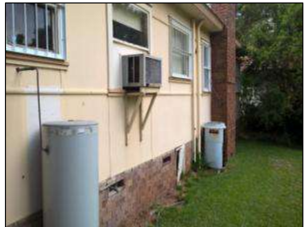
Photograph 5 – Western exterior of subject property in backyard and sub-floor space access.
