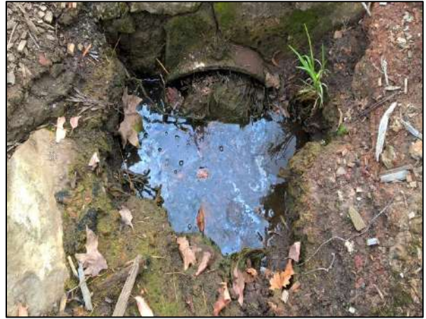
Photograph 10 – Drainage pipe end adjacent to car park with iridescent sheen on water.
