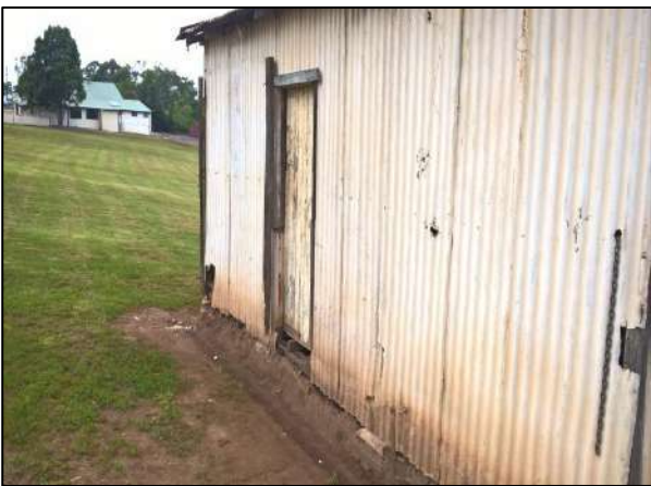
Photograph 8 – Corrugated iron shed with debris on soil surface (facing east).
