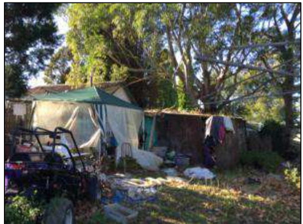
Photograph 12 – Rubbish and garage roof, corrugated asbestos cement roofing
