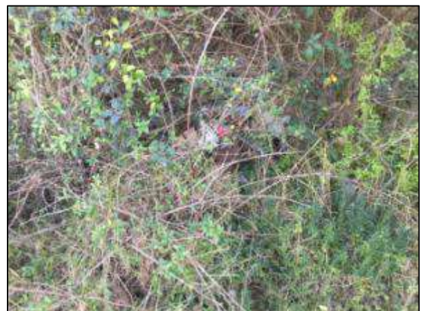
Photograph 6 – Presumed asbestos cement debris located adjacent to the eastern carpark
