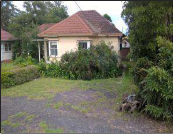
Photograph 1 – Capped front parking area (facing west).
