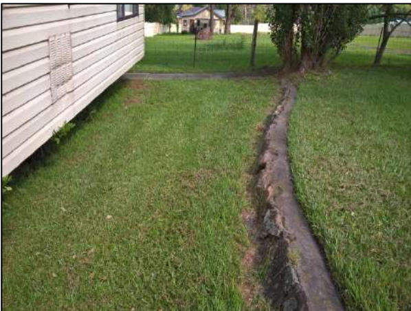
Photograph 5 – Raised border of previous hardstand area indicating cut and fill (facing west)
