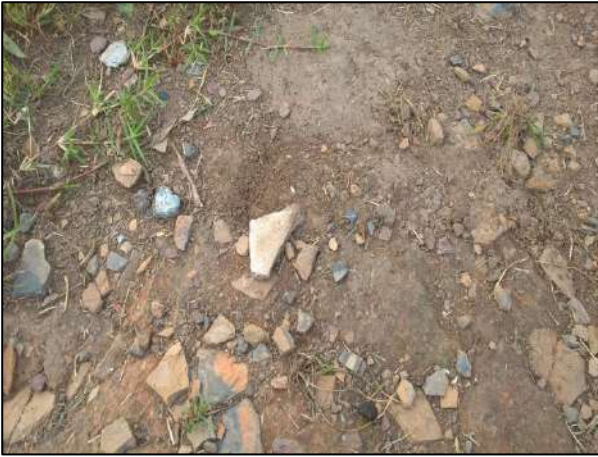
Photograph 7 – Presumed asbestos fibre cement debris adjacent to shed
