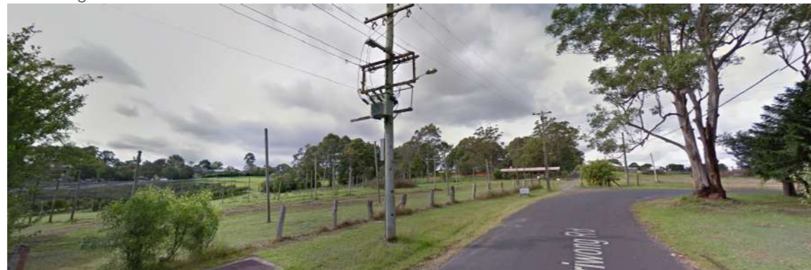
Figure 12: View 2: Eastern view towards subject site on Derriwong Road at bend
