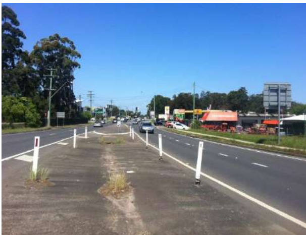
PICTURE 3 – THE OLD NORTHERN ROAD VIEW SOUTH WITH COMMERCIAL PROPERTIES LEFT
