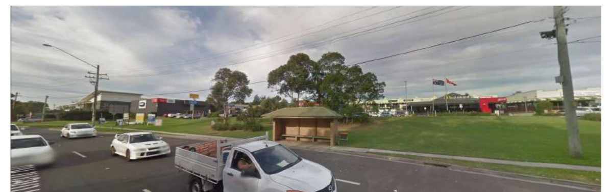
Figure 18: View 8: Towards the edge condition of Dural Business Par.k. Generally, wide separations from boundary to building line decrease perception of safety for pedestrians. Setbacks with building edges closer to the road allow for greater passive surveillance.
