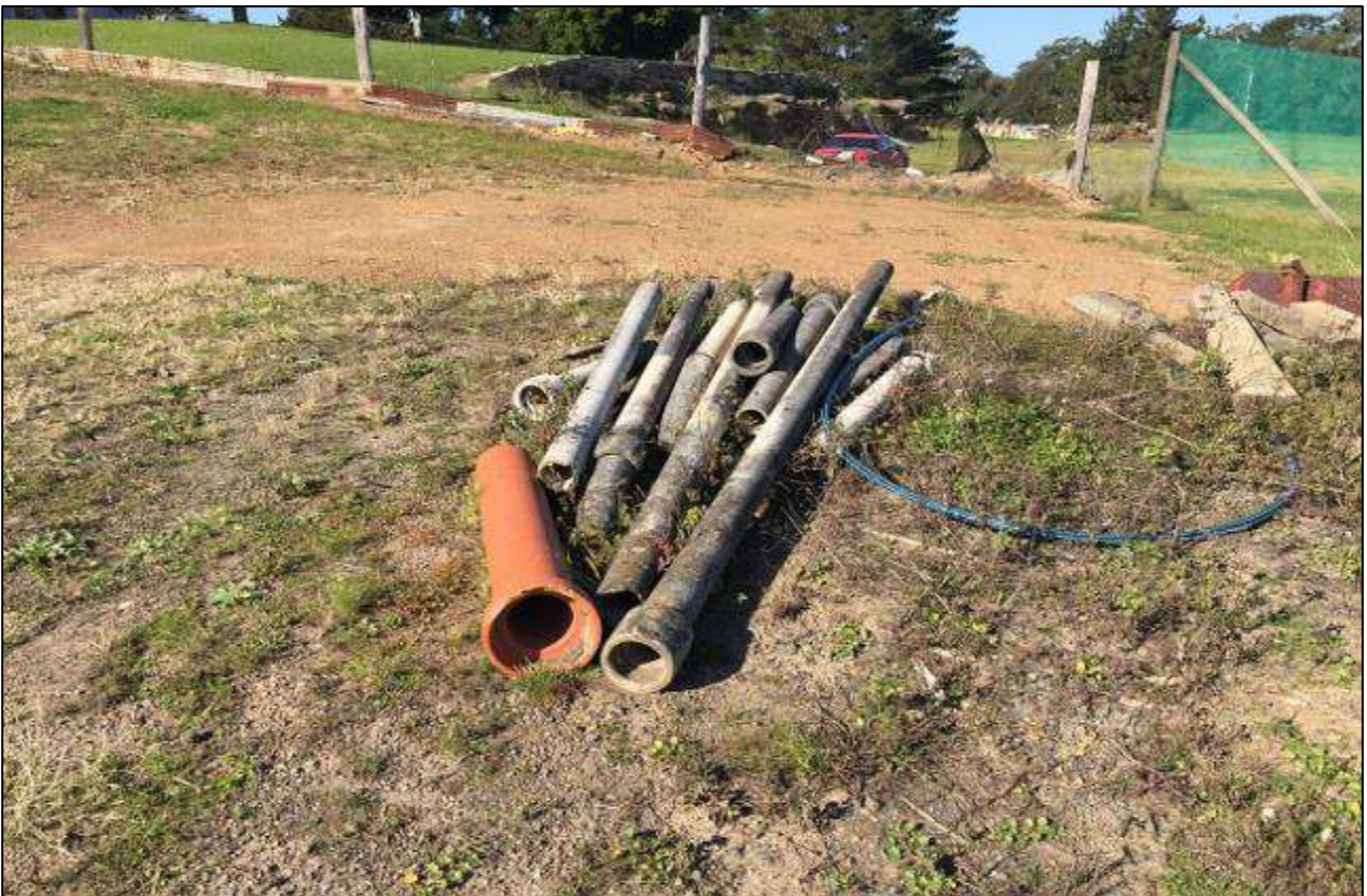
Photograph 8 – Presumed asbestos containing conduits on the eastern storage area of the site
