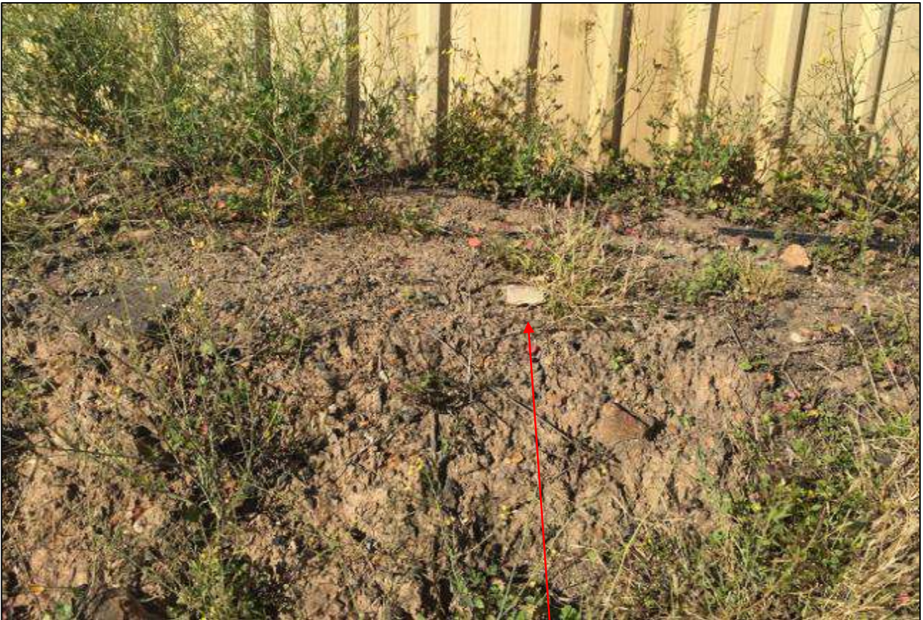
Photograph 2 – Asbestos observed on the surface of the fill material beneath the storage shed.
