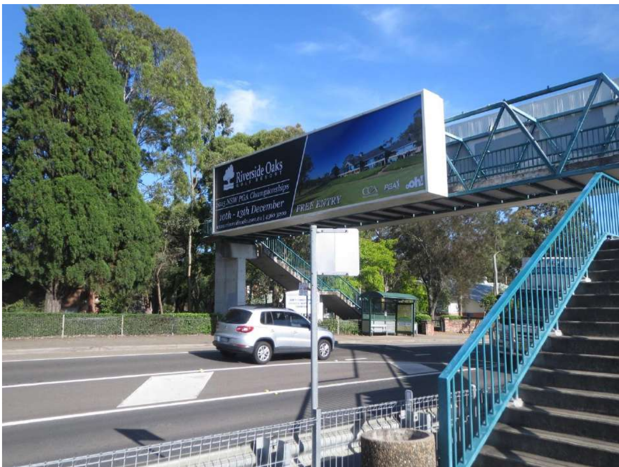
Figure 3 Pedestrian over pass
