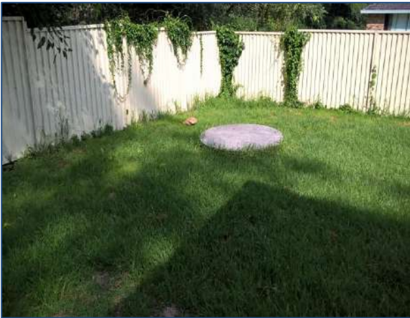
Photograph 3 – Septic tank with disturbed soil profile in south-western corner of eastern portion
