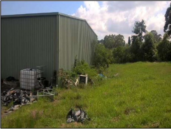
Photograph 7 – General waste surrounding the shed on the northern boundary.
