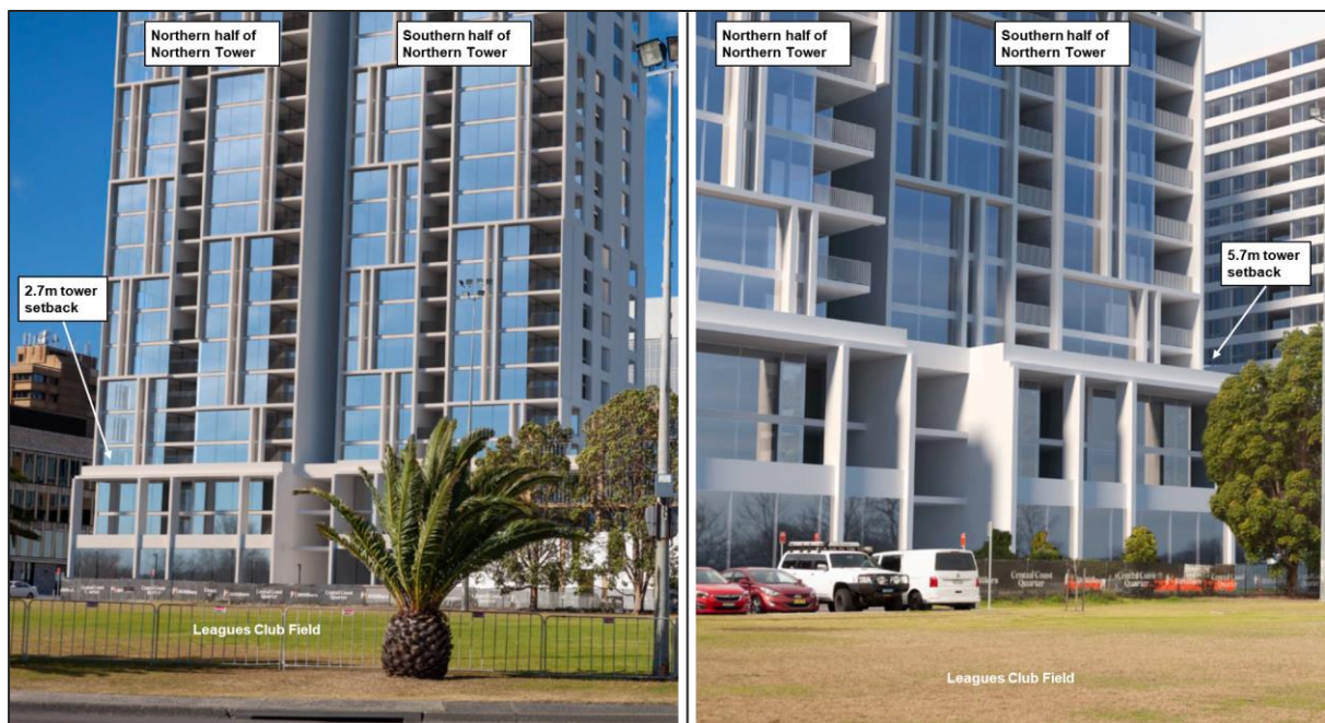
Figure 23 | Perspectives looking from Leagues Club Field to the Northern Tower, its setback and podium (Base source: Applicant's RtS)
