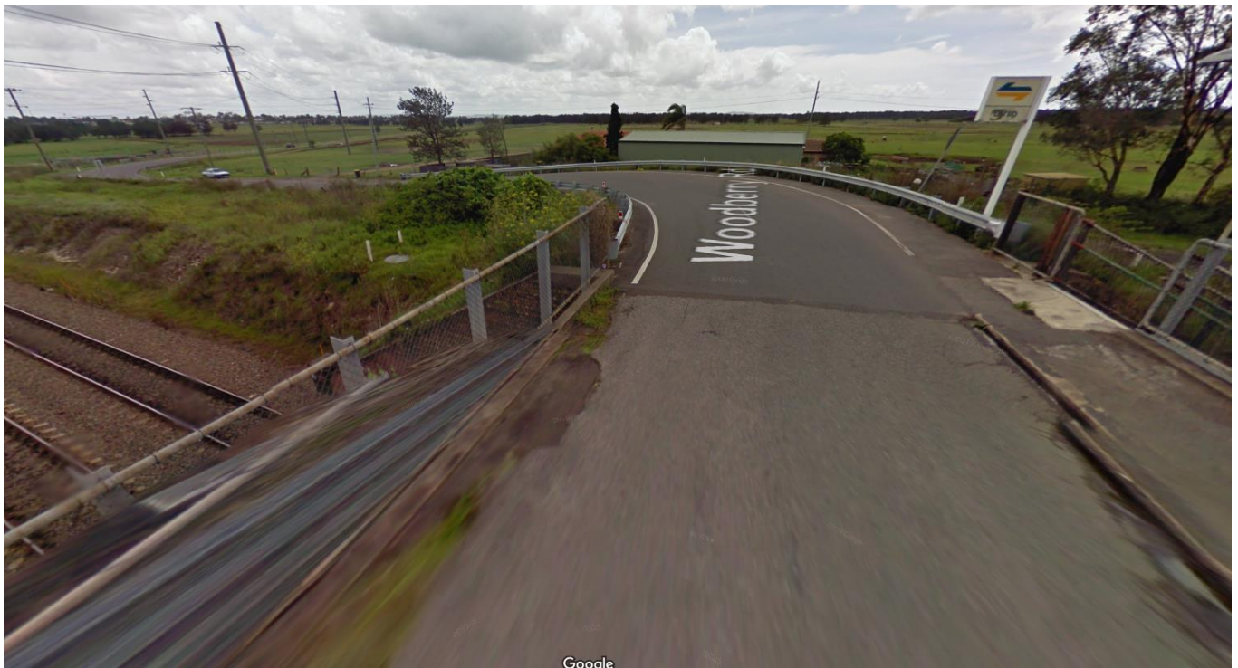
Fig 4: The northern approach to the Tarro railway bridge.
