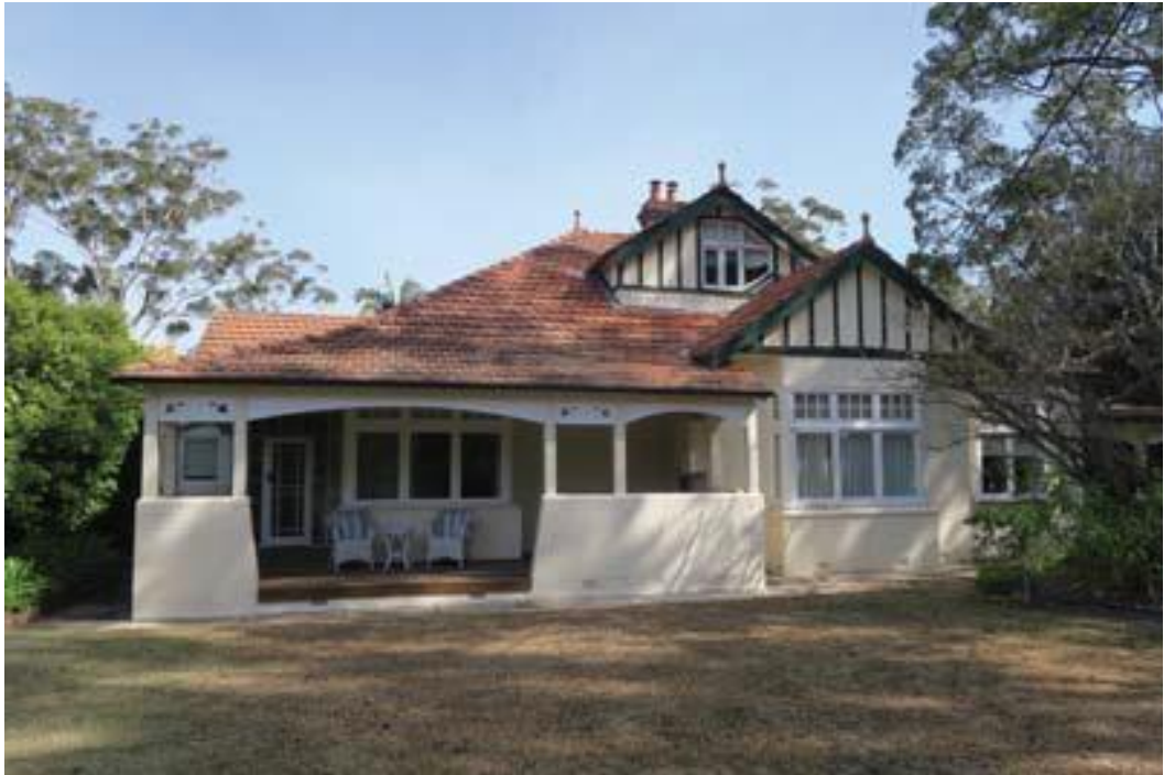
Figure 3: Front elevation of 149 Livingstone Avenue, Pymble (source: Anne Warr heritage assessment report).
